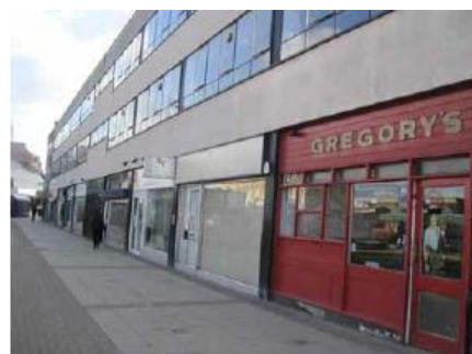
Station Hill Retail Units
