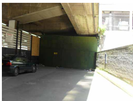
Entrance to Underground Car Park
