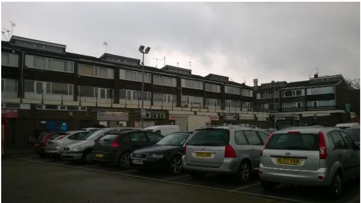
Figure 16: B3 and B4 with adjacent car park.
