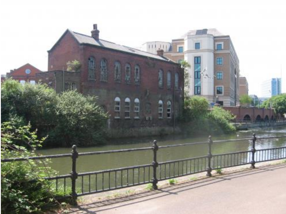
The application site
