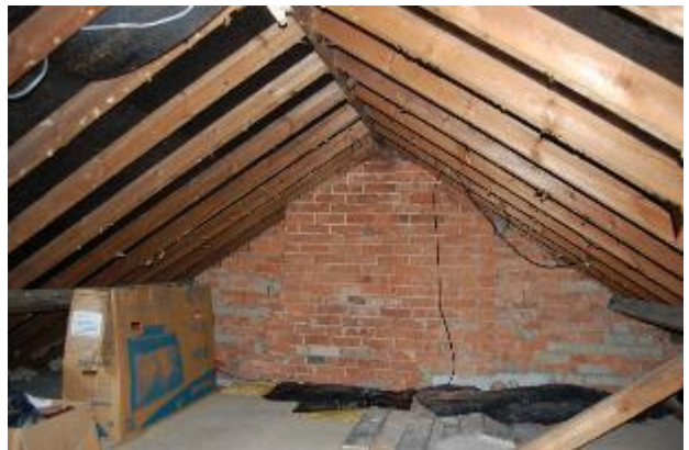
Photograph 6. The loft space within the dwelling.
