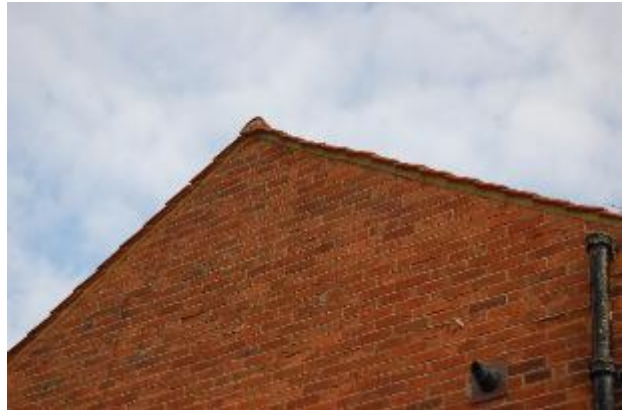
Photograph 4. A photograph showing the excellent condition of the brickwork.
