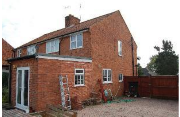
Photograph 2. The south-western gable end of the dwelling to be affected by the proposed extension.
