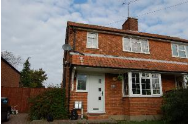
Photograph 1. The south-eastern elevation of the dwelling (123 Peppard Road).
