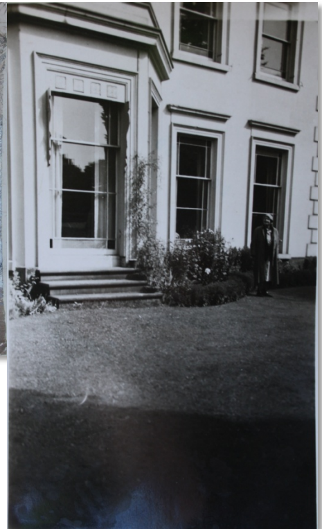
Detail of the bay window to the west elevation
