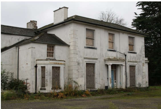
Front (north) elevation of the House
