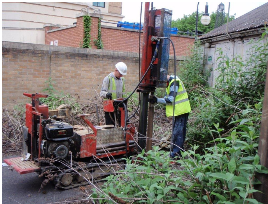
Photo 1: Drilling rig and crew.
