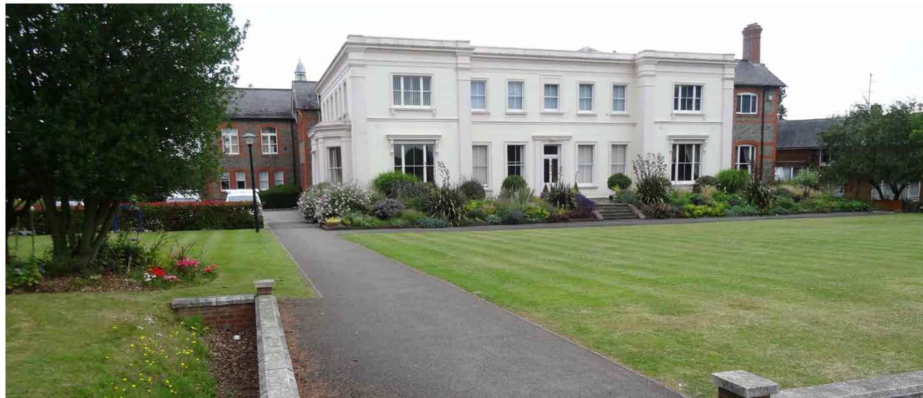
2. South Elevation of Old School
