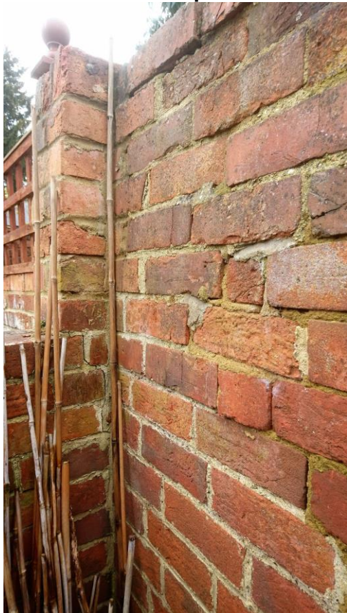
Pillar to the left – part of the wall
