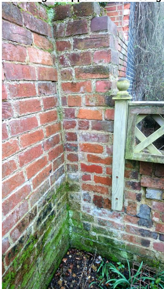
To the right support from existing wall
