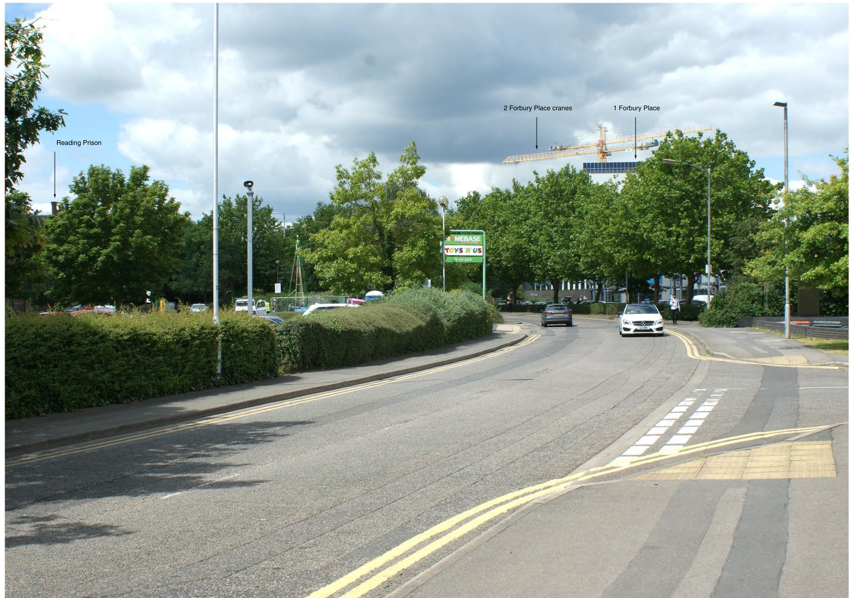
From Kenavon Drive Taken near the entry road to McDonalds.
