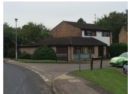
Extensions to no 1 Chatsworth Close
