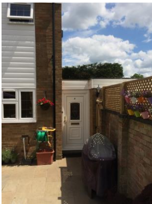
Rear Entrance (Via rear garden)
