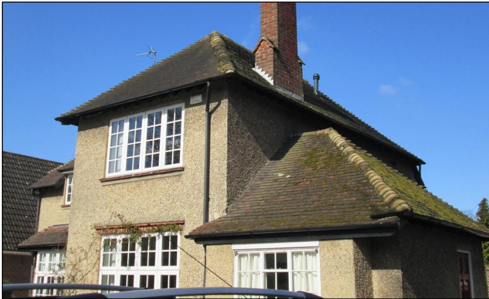
Figure 4 – North-eastern (side) elevation, showing single storey extension
