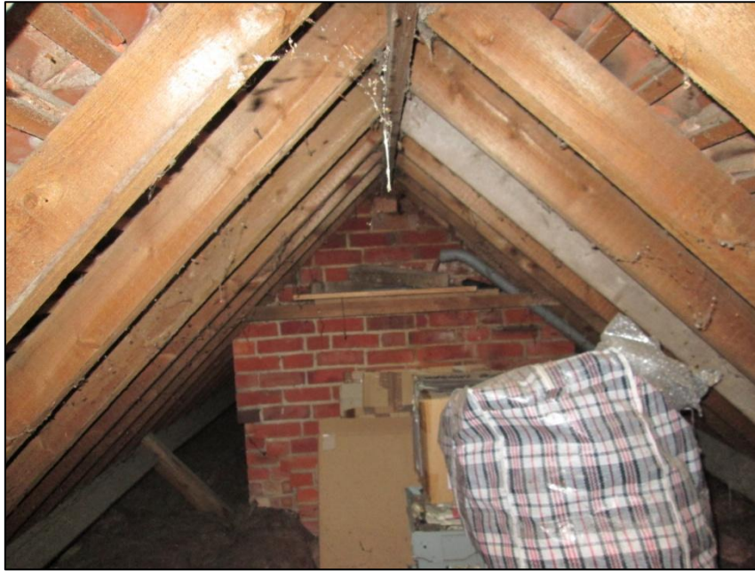
Figure 5 – Chimney stack located towards the southern end of the property
