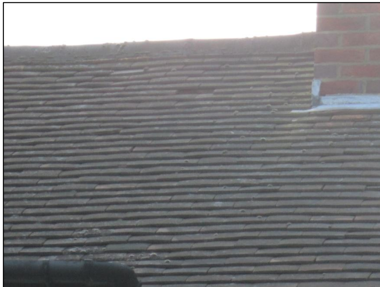
Figure 10 – Tile roof covering showing good condition with only a couple of lifted tiles
