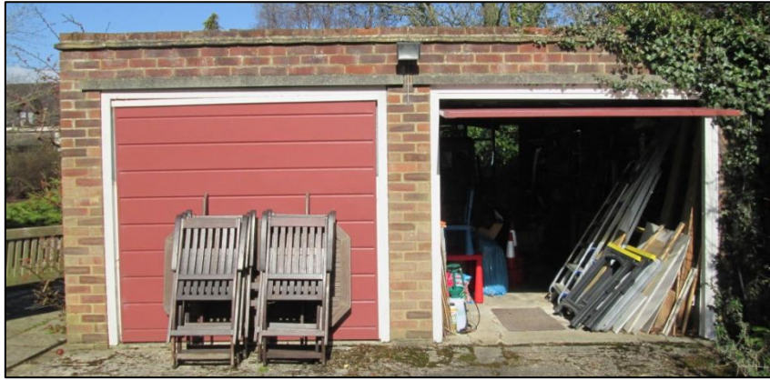
Figure 7 – Exterior of the double garage, showing brick construction, doors and flat roof
