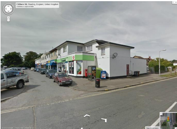
View of the Front of the Store (Google Streets)
