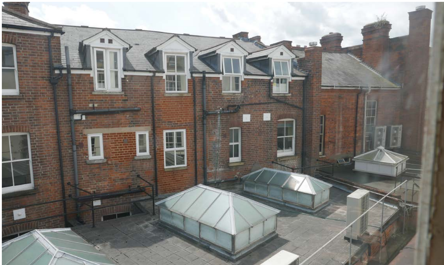
1960's extension with bulky modern rooflights
