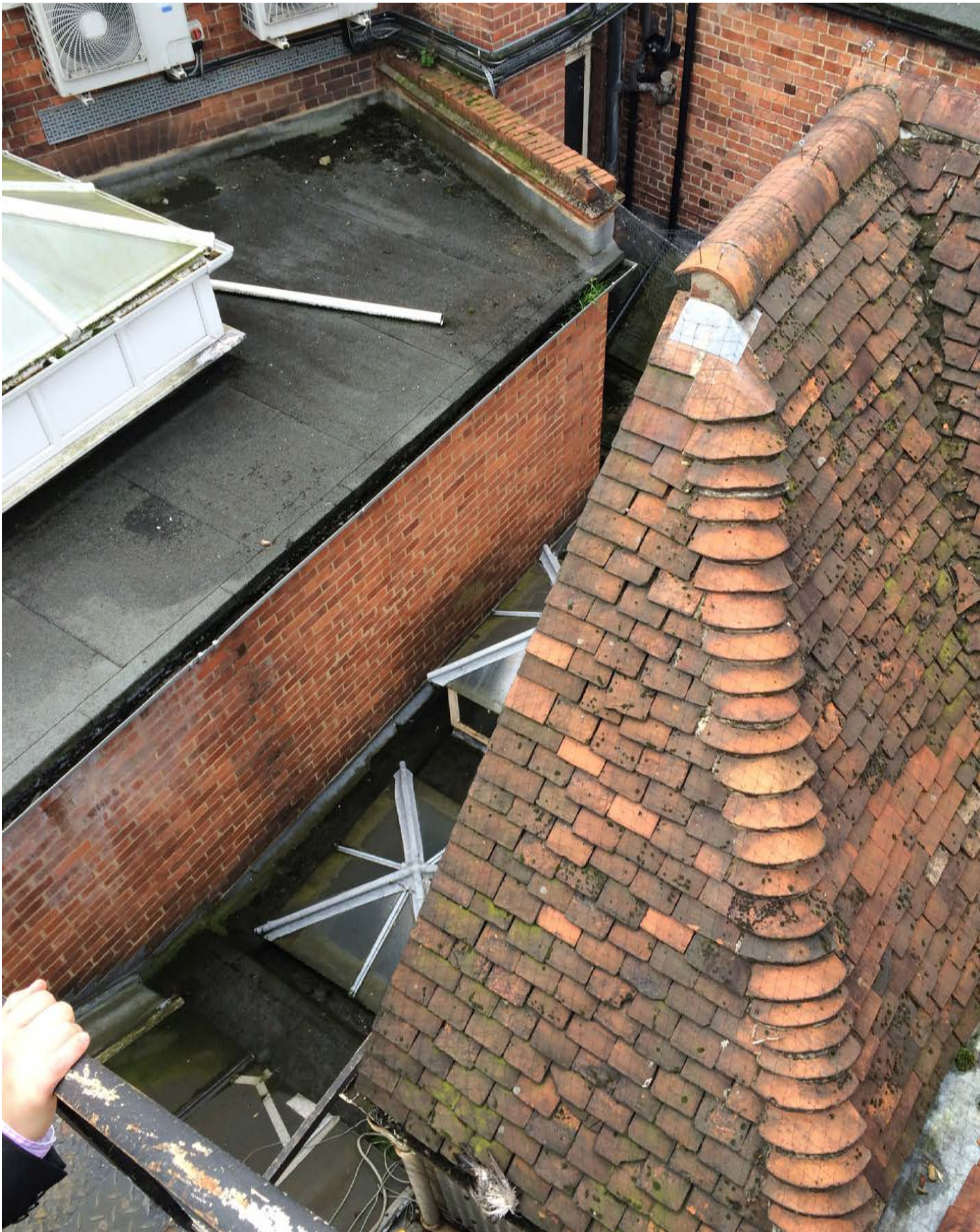
Ad-hoc roofscape at rear of Jacksons
