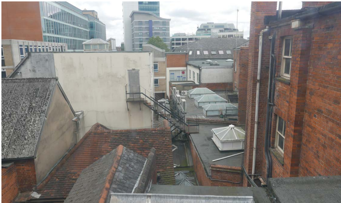
Various ad-hoc structures at rear of Jacksons
