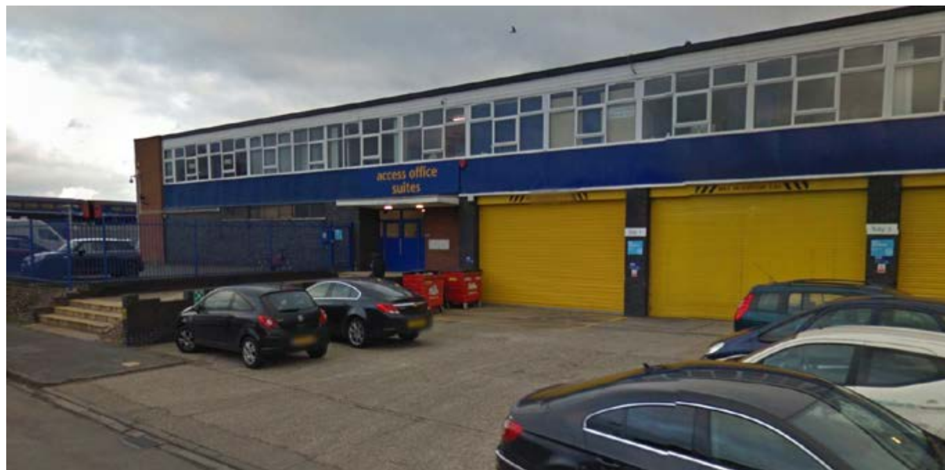
Photo 4 View to entrance to office suites & self storage loading bays
