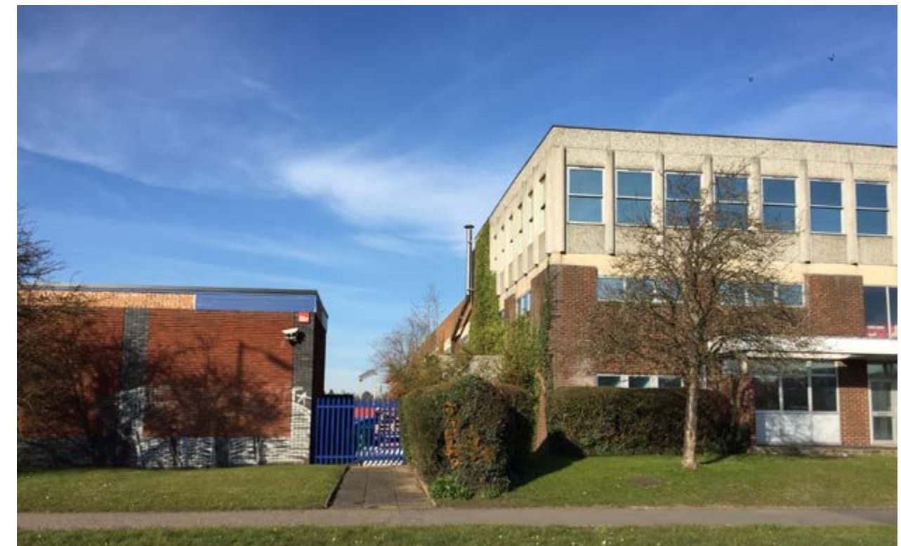
Photo 8 View of East end of front facade and neighbouring property
