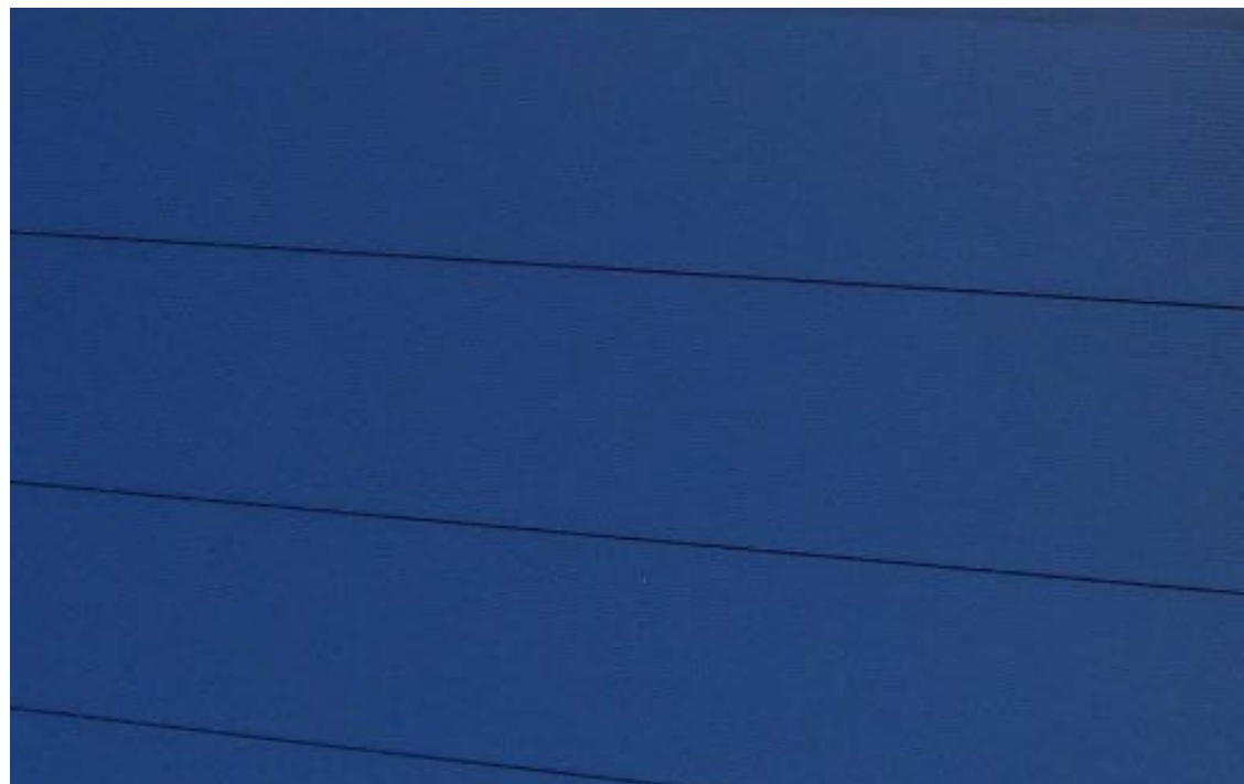
Silver, mid grey and blue microrib cladding panels to the primary elevations.
