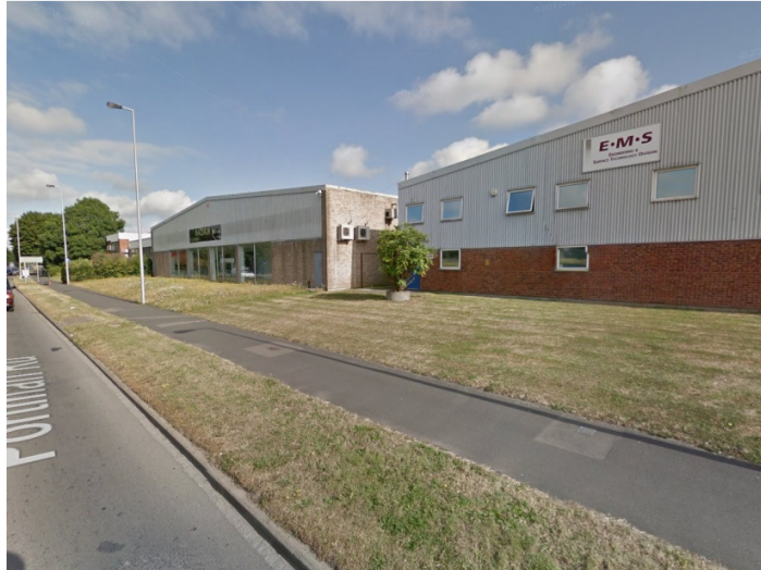
View of the existing showroom from Portman Road
