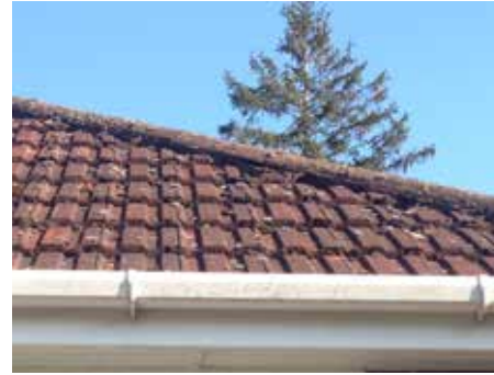
Plate 3: Gap under ridge tile providing potential roosting feature
