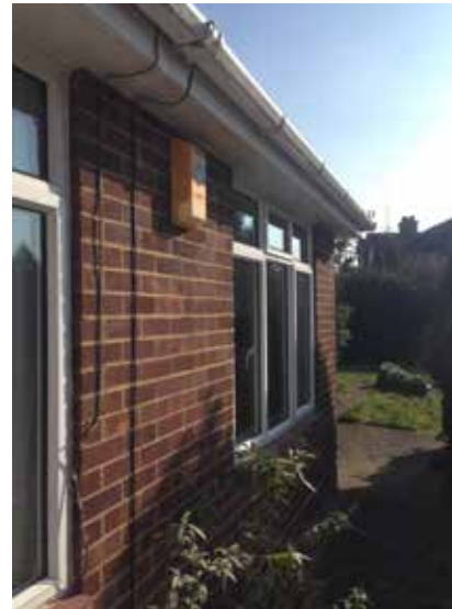
Plate 4: Modern PVC soffits in good condition and affording no opportunities for roosting bats.
