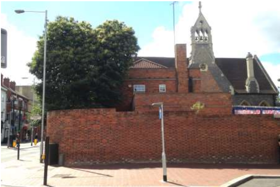
Figure 34: View of the Quadrant Walls on the corner of Friar Street and Greyfriars Road.
