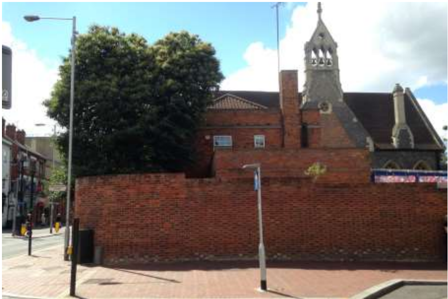
Figure 26: View from adjacent to the western elevation of Central Studios towards Greyfriars Church and the Quadrant Walls.
