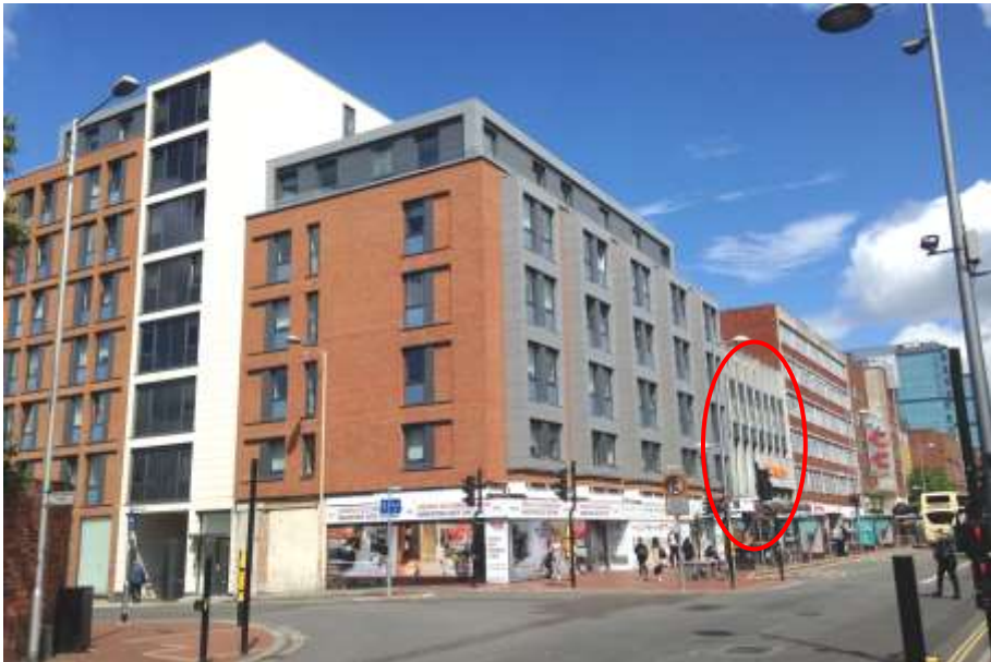
Figure 27: View from the junction of Friar Street and West Street towards the Site (marked in red).
