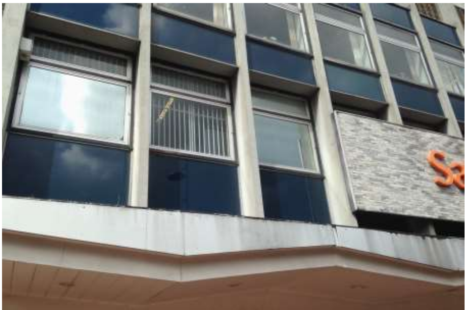
Figure 20: Close-up of southern elevation.
