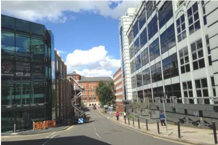
Figure 31: View looking south along Greyfriars Road adjacent to the rear of the Site towards Station Hill.
