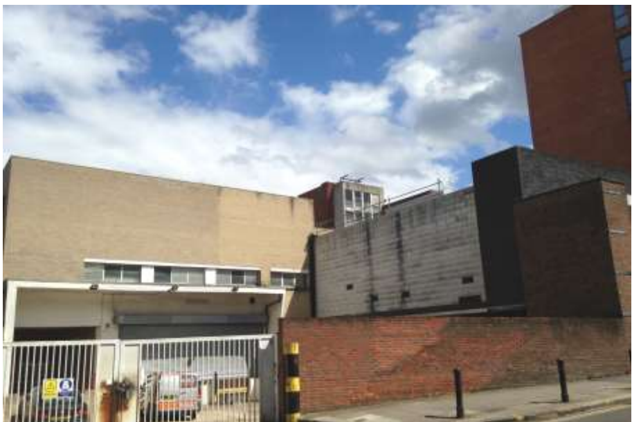
Figure 22: Rear loading facilities and storage to the rear of the Site as seen from Greyfriars Road.
