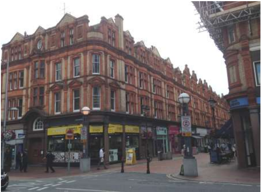
Figure 38: Queen Victoria Street.
