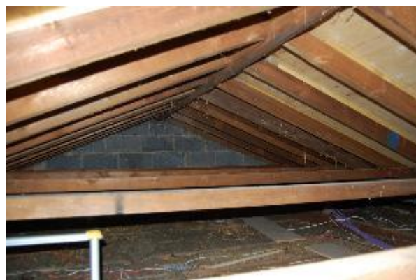
Photograph 2. The loft space of Building 3.
