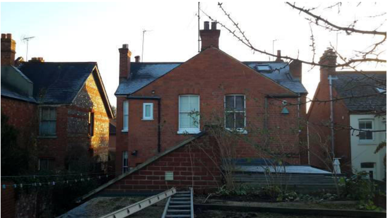
Photo 01. General view of the rear elevation
