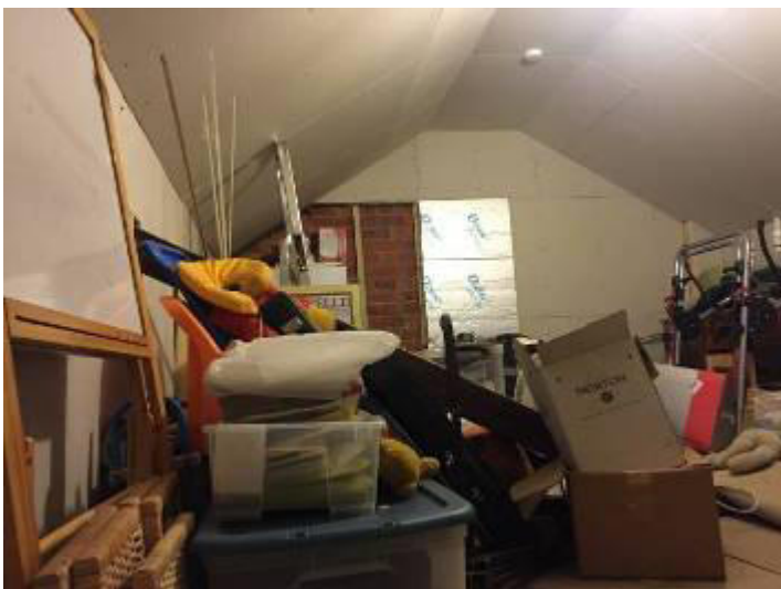
Photo 03. General view of the attic.
