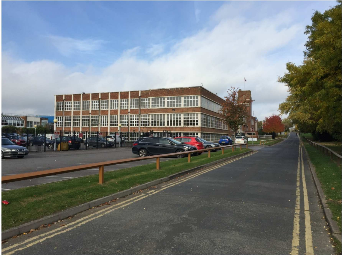
Front elevation viewed from the south east
