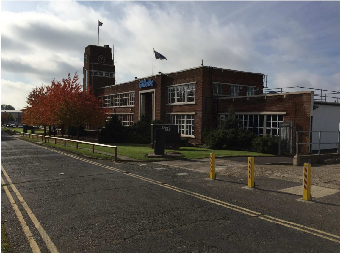
Front elevation viewed from the north east
