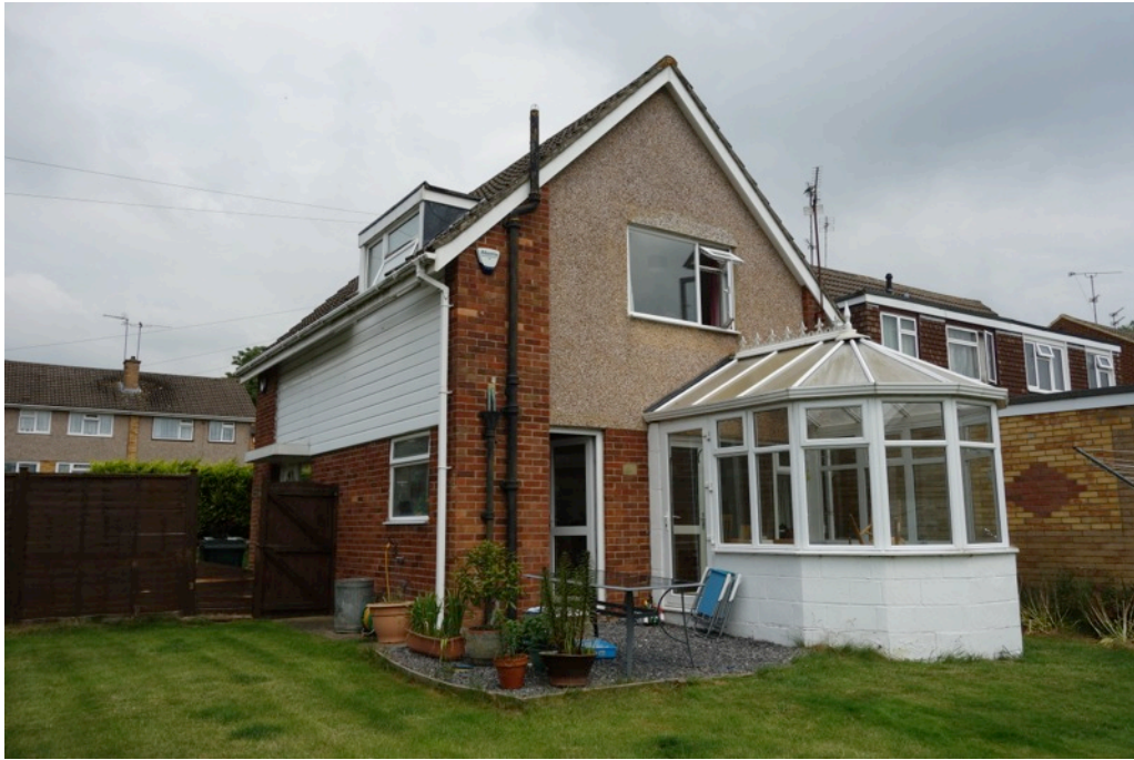
1 Hay Road south west elevation, conservatory to be demolished.
