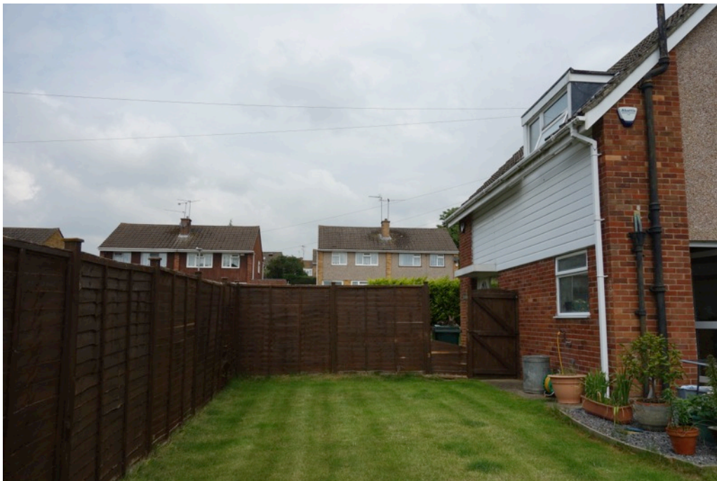
West elevation and garden to the side where the proposed extension is to be located
