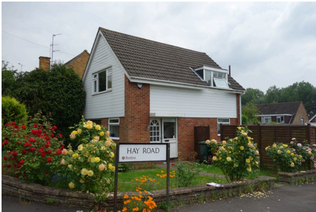
1 Hay Road, north west elevation viewed from the road.
