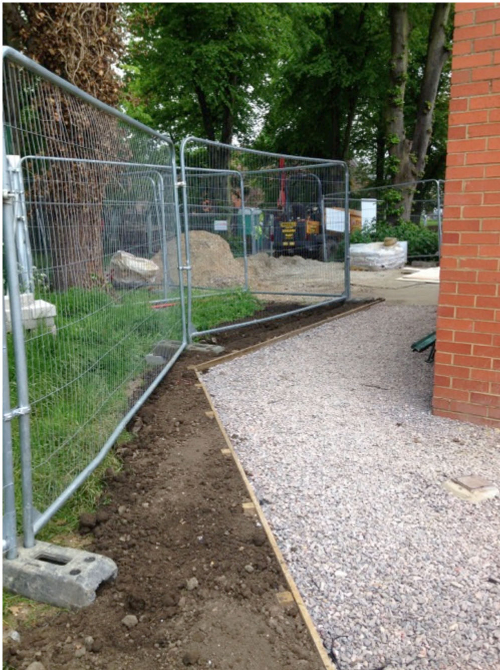
New pathway created using No-dig construction within Root Protection Area of T24. Permeable surface still to be laid.
