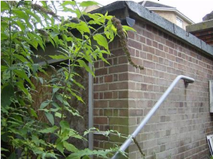
Photograph 4: Building 2 and a small out-house by site entrance.
