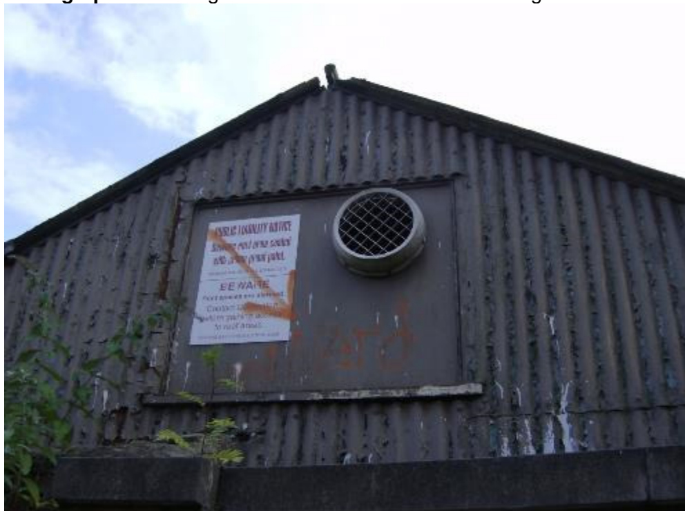
Photograph 8: Building 5 – vent on western side of building.
