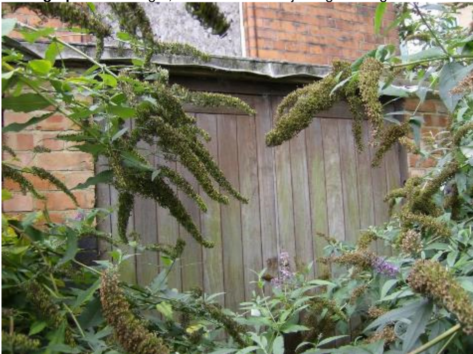
Photograph 6: Building 3, a small lean-to adjoining building 1.
