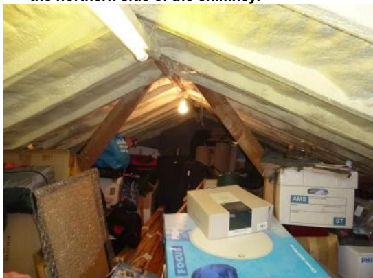
9. Internal view of the pitched roof.
