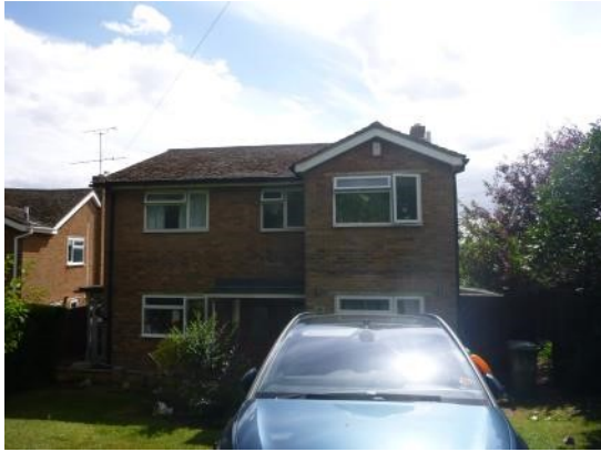
1. The front of the property viewed from the north.
