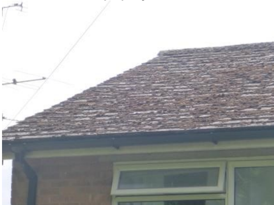
3. Tightly fitted roof and ridge tiles.
