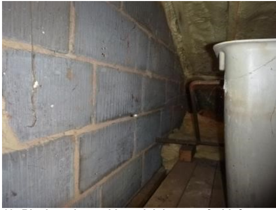
13. Block work at gable end tight to roof with foam insulation.
