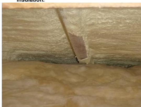
12. Eaves filled with foam insulation.
