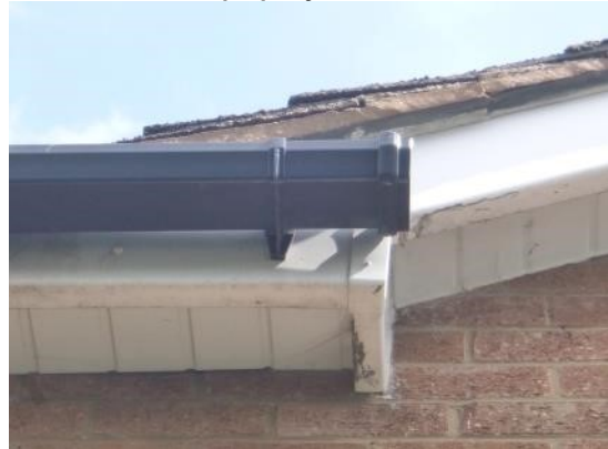
4. Mortar in place at the eastern facing gable end.
