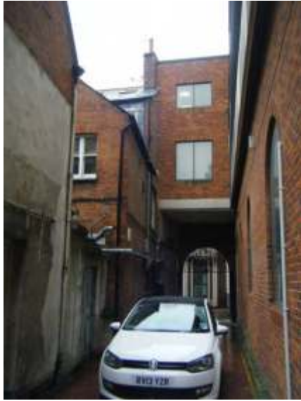
Appendix 4.5: View west within alleyway.
