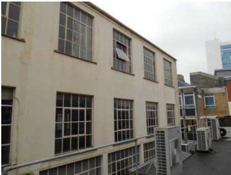
Appendix 4.7: View to rear of Jacksons warehouse.
