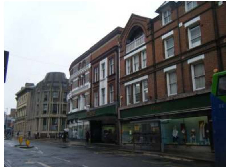
Appendix 4.4: View west at Jacksons Corner.
