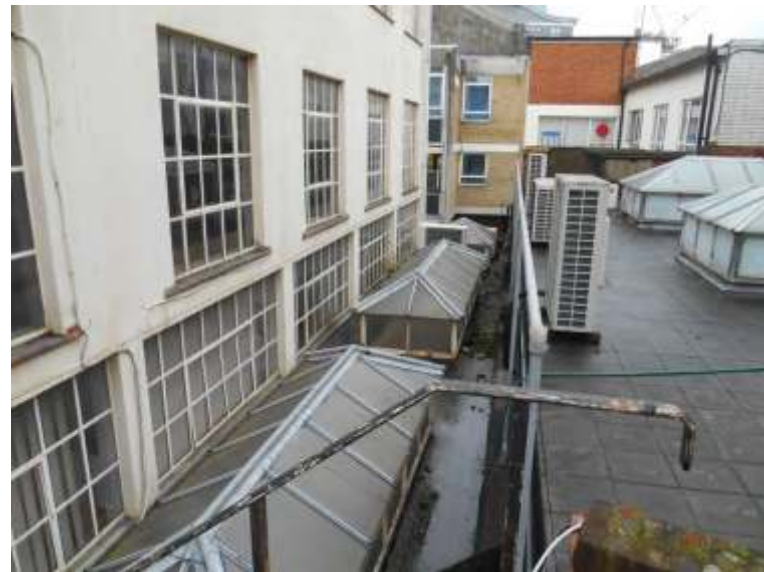
Appendix 4.8: 1936 warehouse to the rear.
