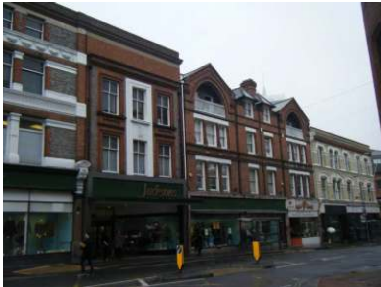
Appendix 4.3: Jacksons building along King's Road.
