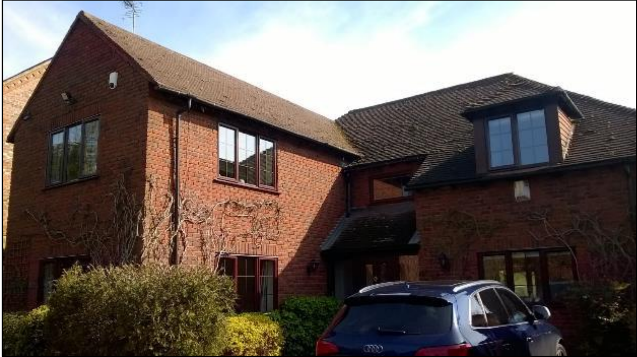
Photo 1: The southern and western elevations of B1.
