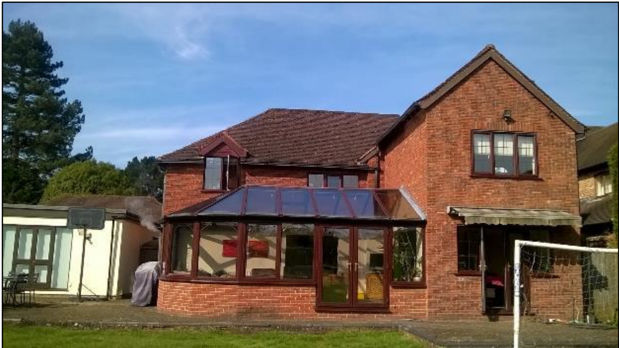
Photo 2: The eastern elevation of B1.
