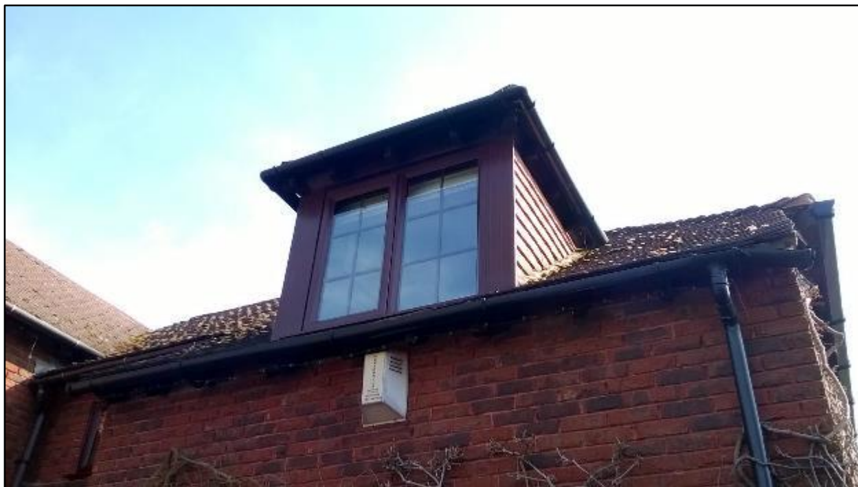
Photo 3: The western elevation dormer window of B1.
