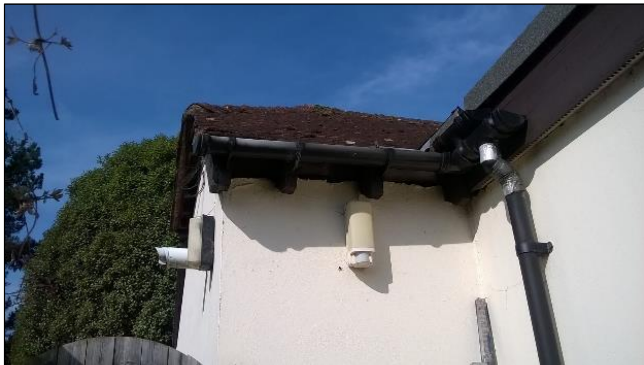
Photo 11: The pitched roof and flat roof of B2.
