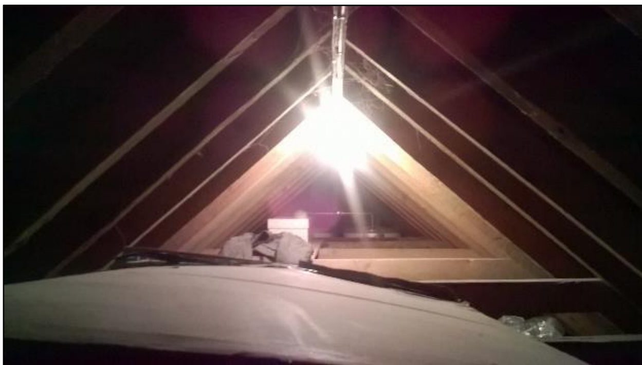
Photo 6: Loft space of B1.
