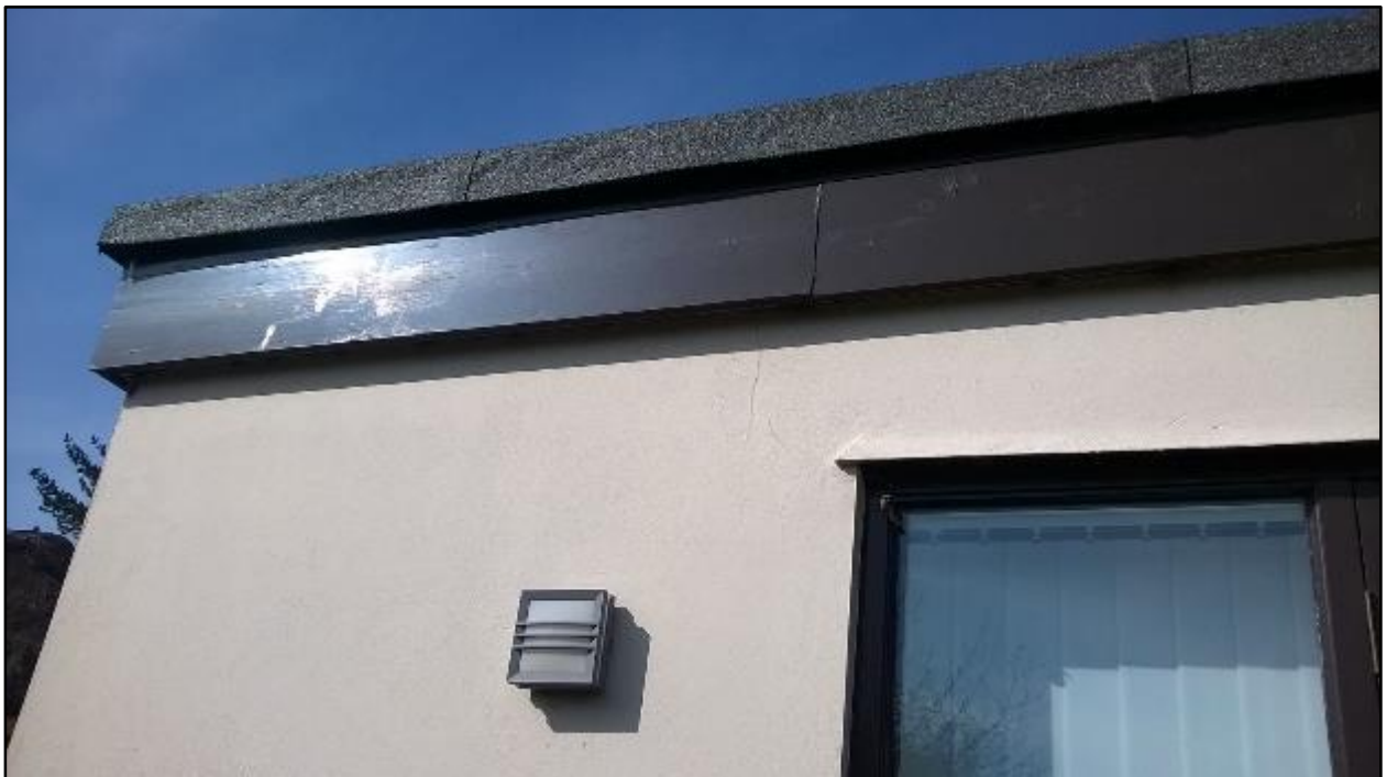
Photo 10: The timber boards across the elevations of B2.
