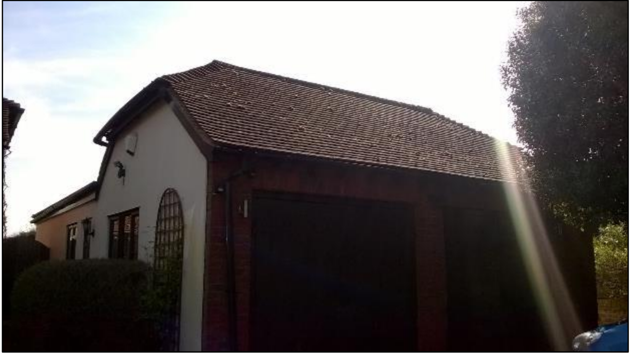
Photo 9: The western and northern elevations of B2.
