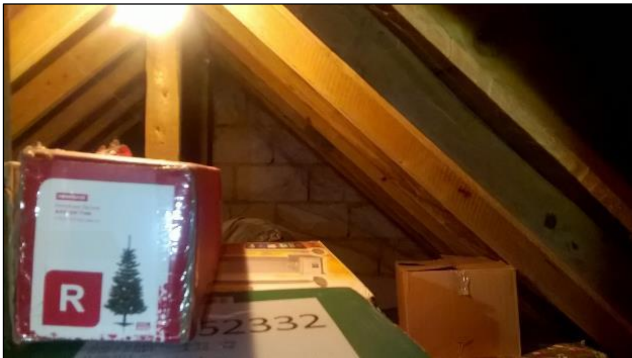
Photo 7: Loft space of B1.
