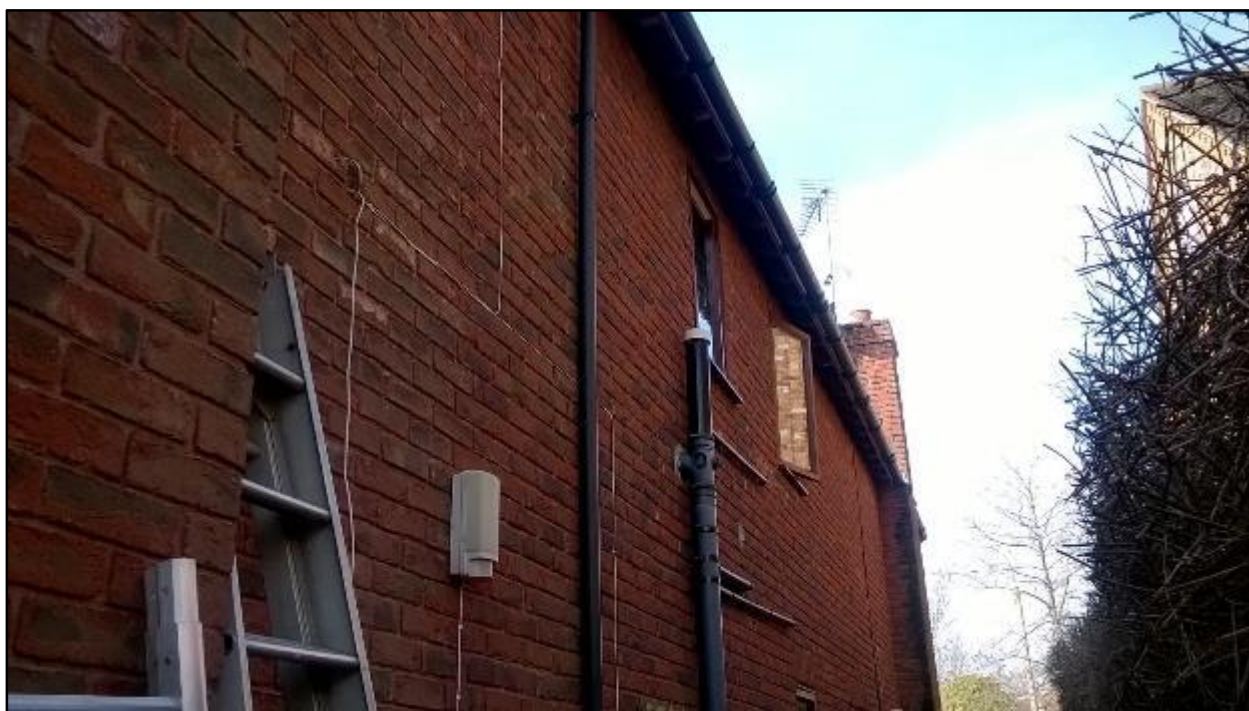
Photo 4: The northern elevation of B1.
