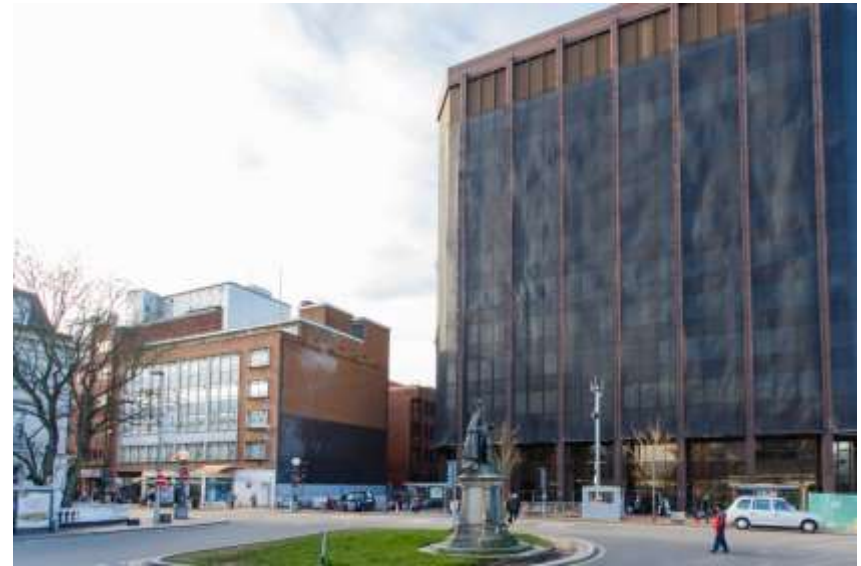
1 – Looking towards 29 to 35 Station Road from Station Approach
