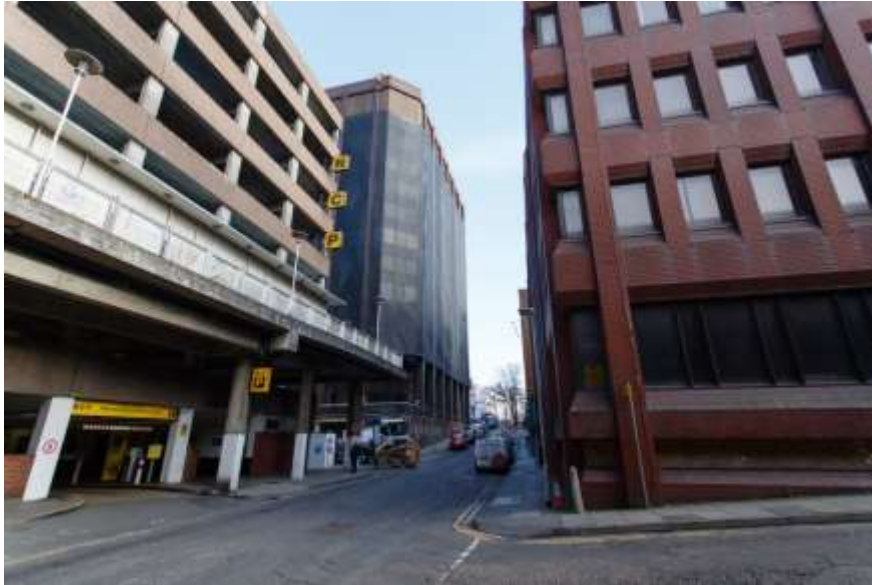
Garrard Street looking towards Thames Tower [Photograph 03/12/14]
