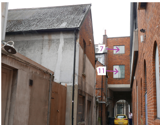
Image showing windows 7 & 11 on 1-2 Market Place
