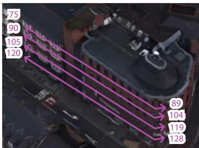
Views of 2-12 Kings Road showing windows 75-135 to the south of the proposed site
