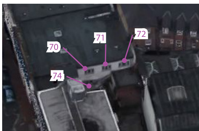
Views of 11-13 Kings Road showing windows 70-72 & 74
