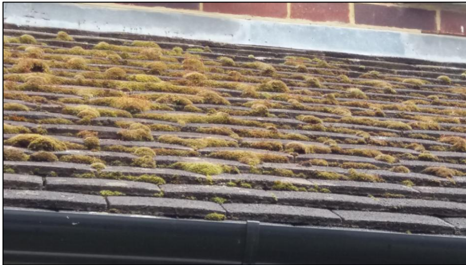
Figure 6 – machine made tile roof covering showing good condition
