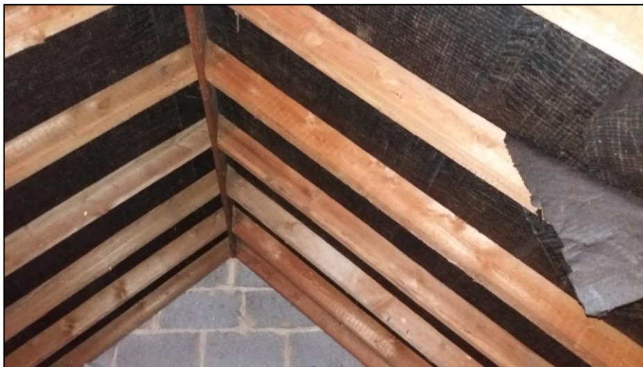
Figure 5 –Bitumen felt underlay was in very good condition
