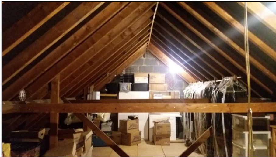
Figure 4 – Roof void showing lighting present
