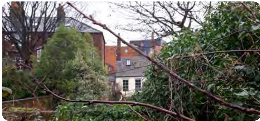
6. Rear view of Rose Cottage to the south of the site
