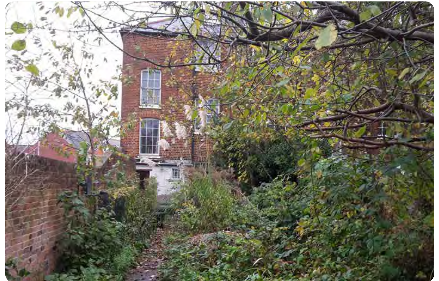
5. View from within site facing back to No.92-96 Southampton Street
