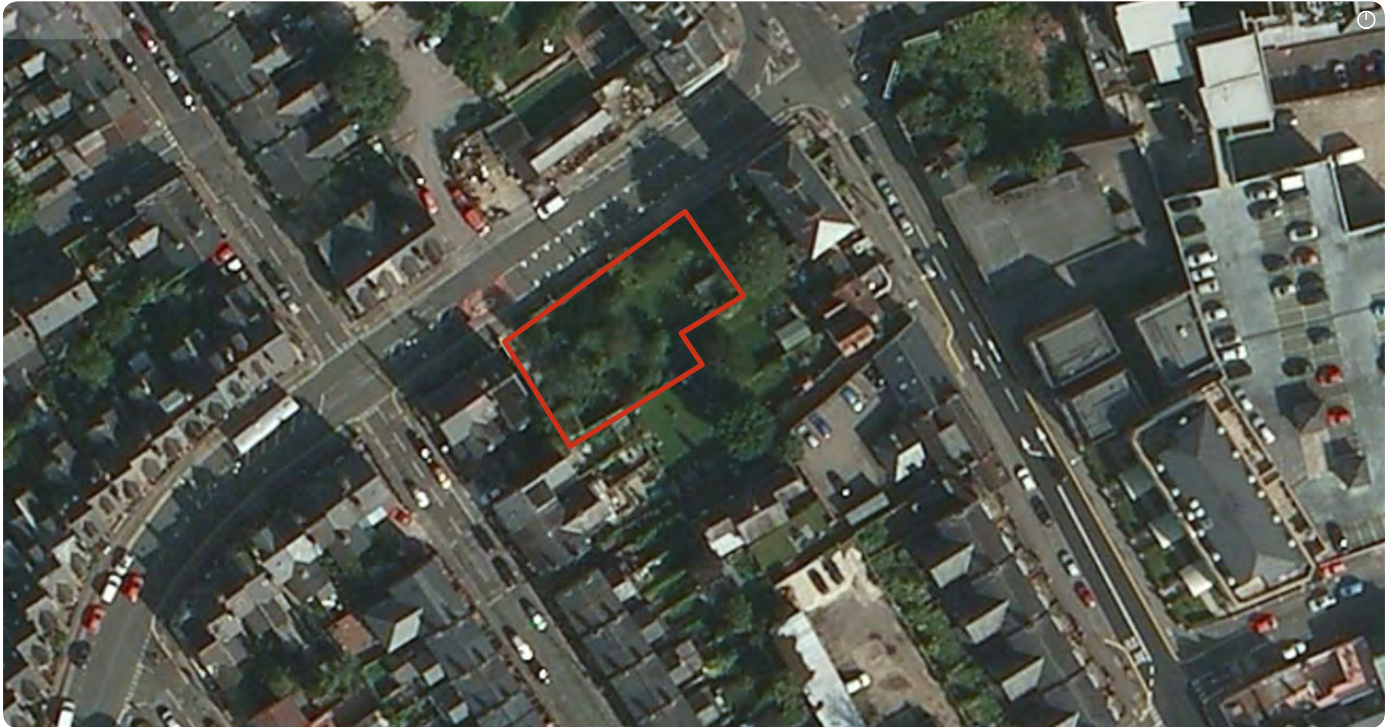
Site location - aerial view
