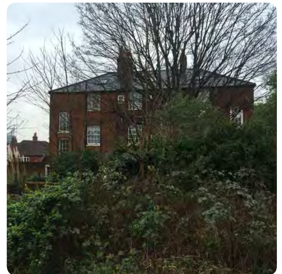
9. Rear elevation of No.92-96 Southampton Street
