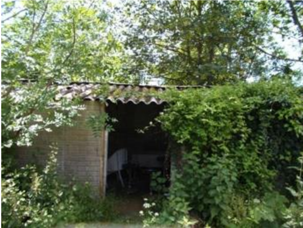
Photograph 5: Prefabricated concrete building with corrugated roof in Area 2
