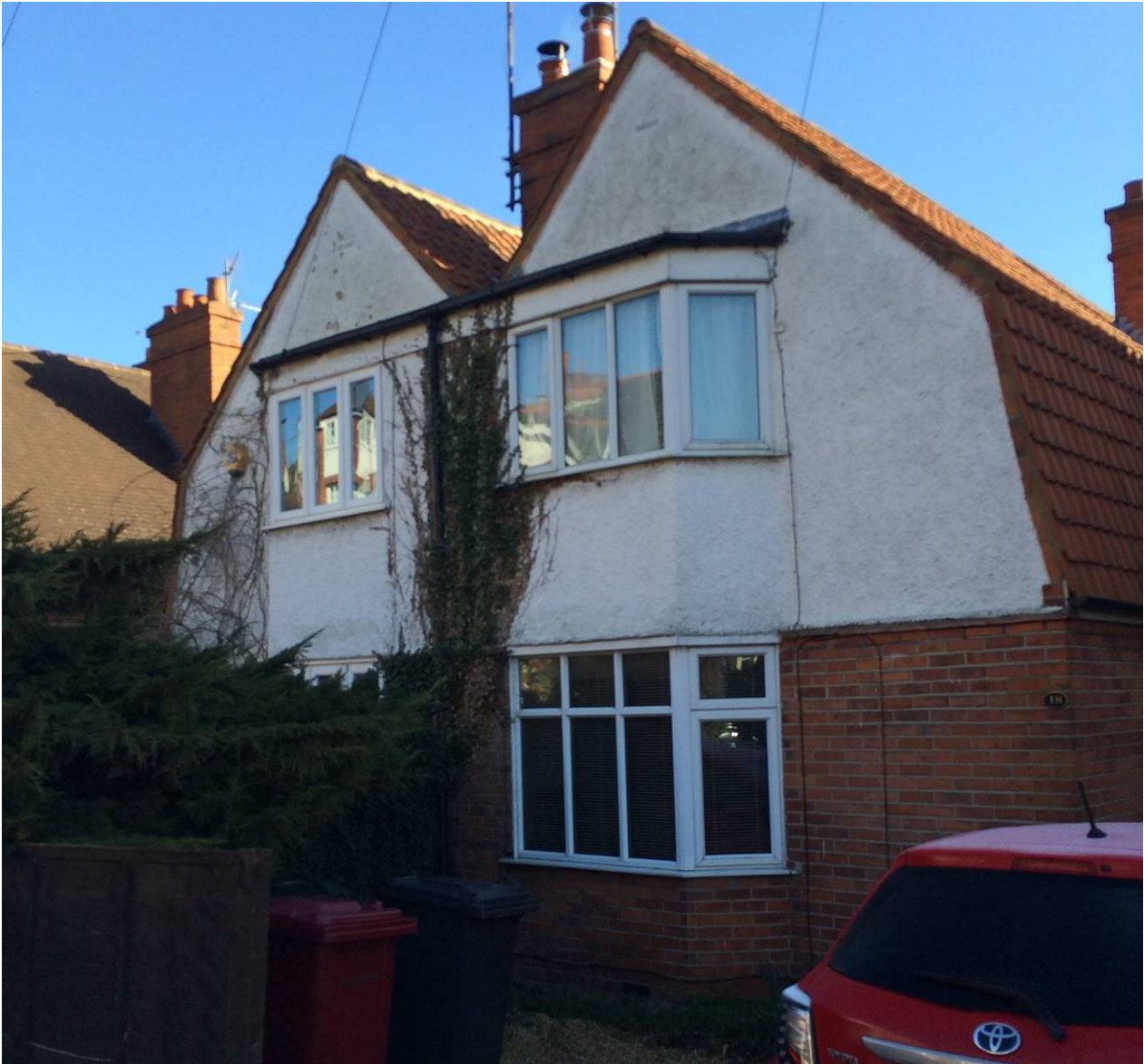
Street elevation from St Anne's Road showing mansard roof form
