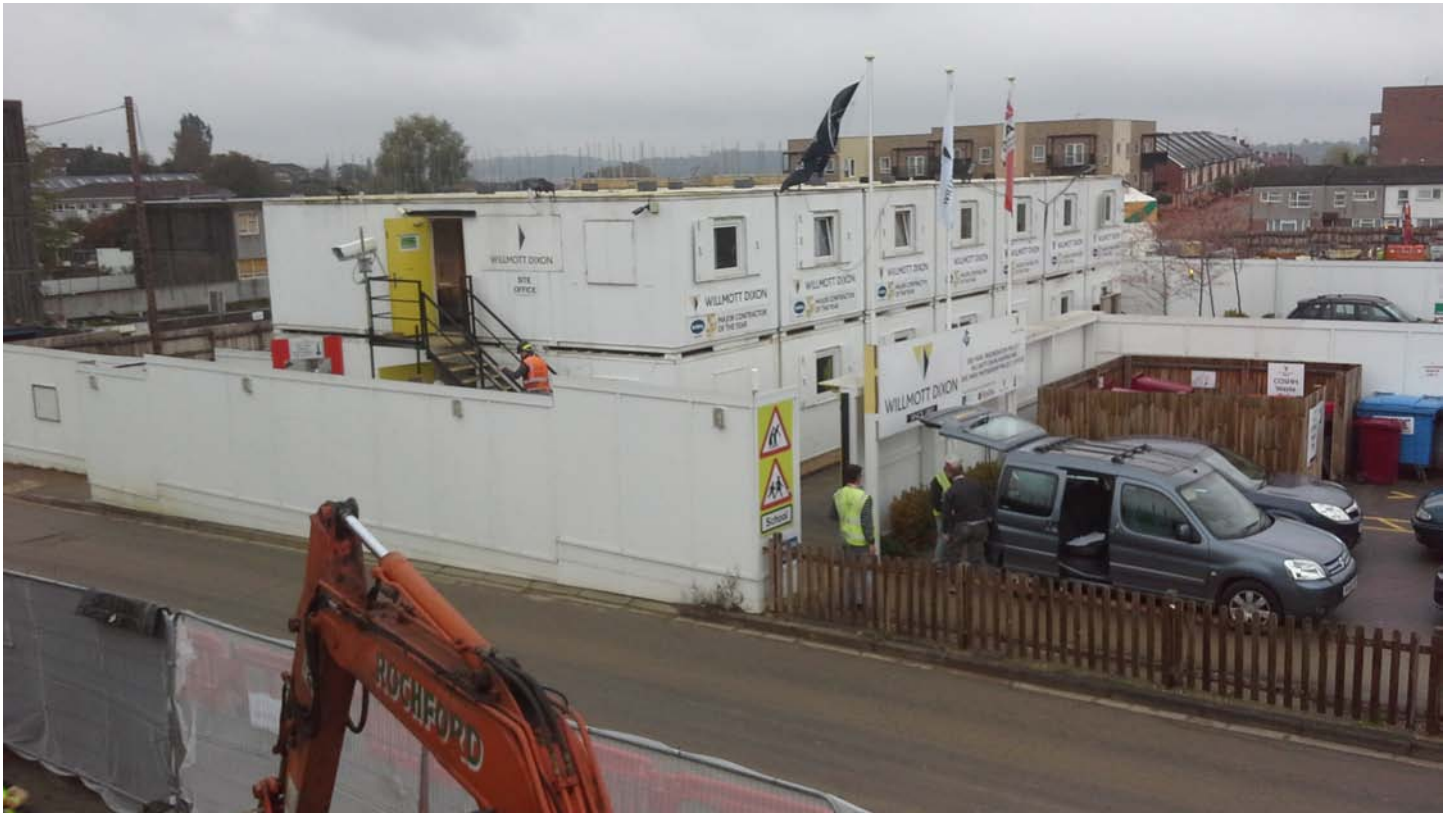
Photo showing the proposed type of modular accommodation units that are to be used to provide the temporary Youth and Police Facility.
