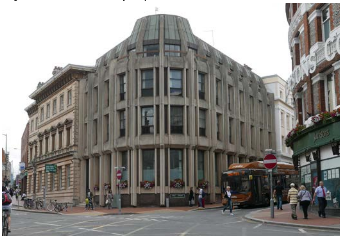
Fig 2.14: View of corner High Street / King Street
