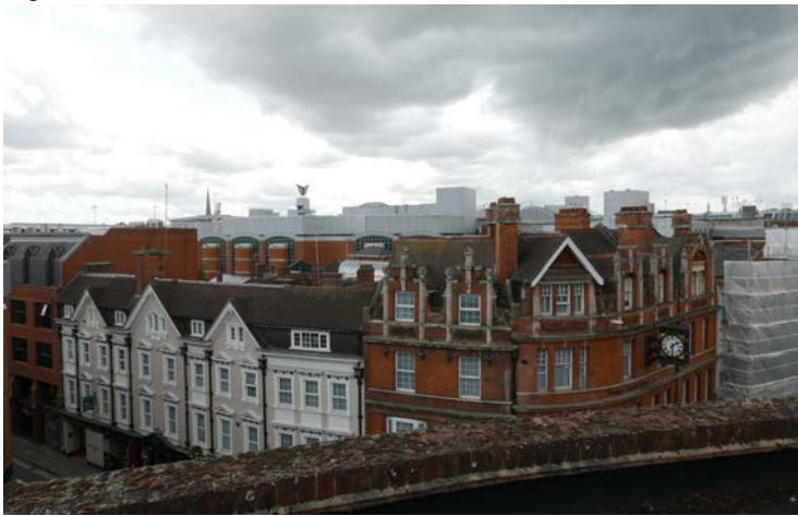
Fig 2.17: View from roof of Jacksons Corner
