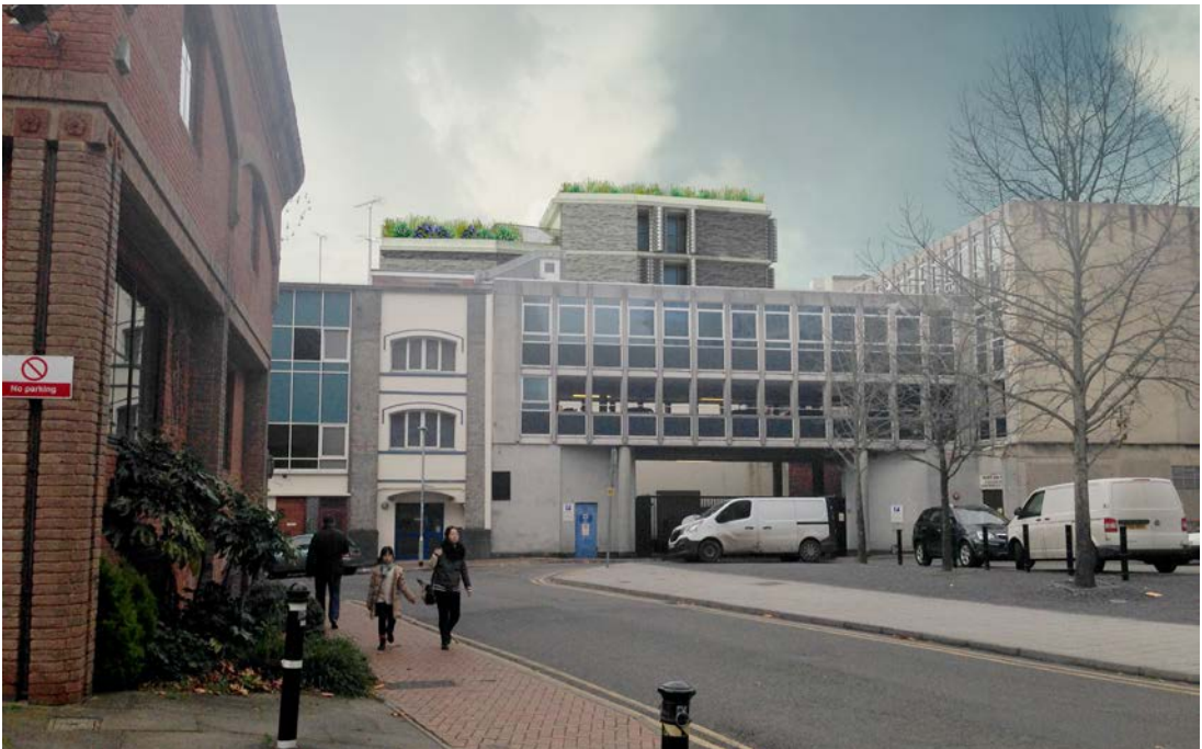
Photo - Abbey Square (not part of the conservation area) - Visible portion will enhance the streetscape
