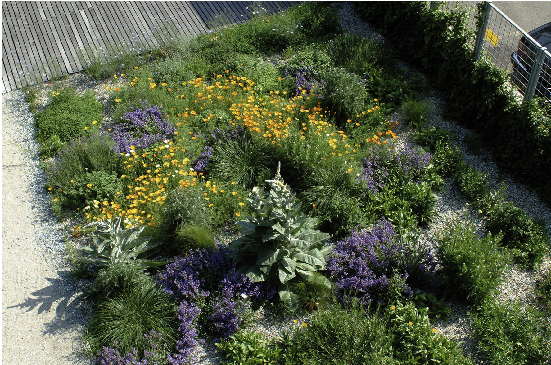
Typical mixed species semi-extensive living roof
