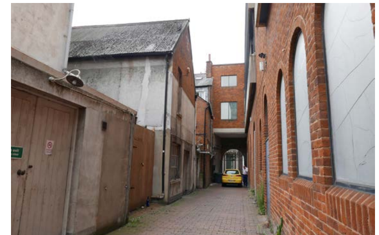
Fig 2.2: Rear Laneway towards High Street
