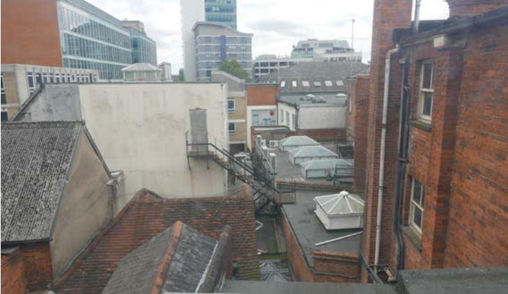
Fig 2.9: Various ad-hoc structures at rear of Jacksons
