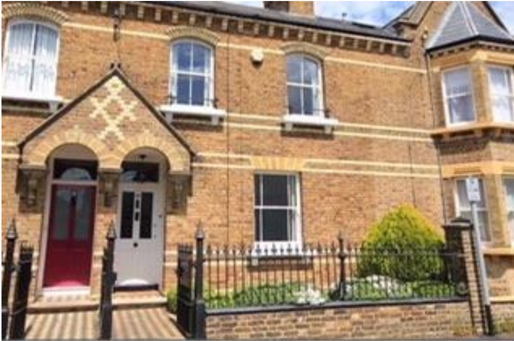
B1: Street Scene and outside front of property, showing the Grad II listed building features in line with neighbouring properties. This is a south facing property.
