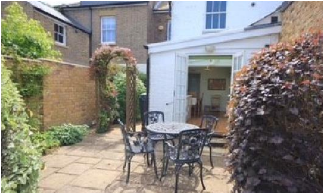
B2: Rear of property. Photo shows the rear access and also 1 st floor bathroom window.
