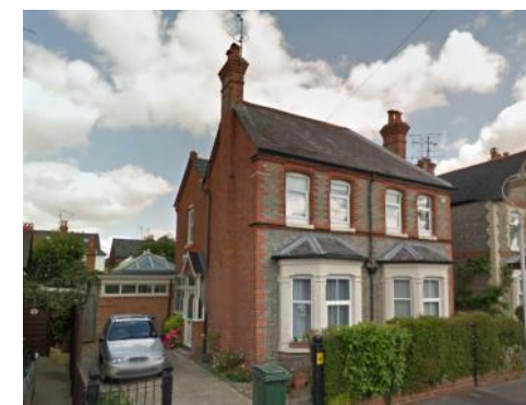
Park Avenue | Brickwork & Plain Roof Tiles
