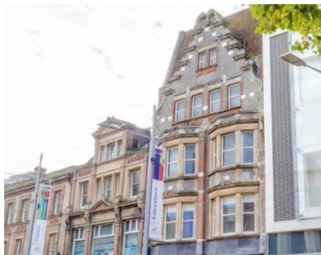
Broad Street | Decorative Gable
