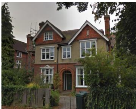
Craven Road | Brick, Pebbledash & Hanging Tiles
