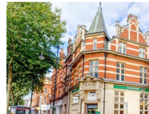
Broad Street | Red Brick & Stone Work
