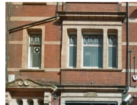
Station Road | Brick & Stone work
