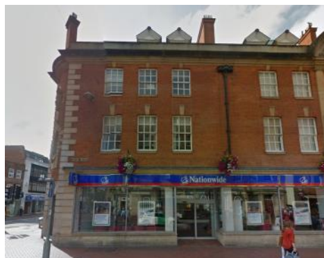
Station Road | Brick, Stone work & Dormers
