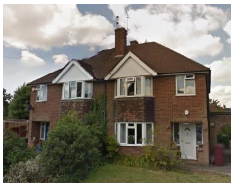
New Road | Brickwork & Tile Hanging
