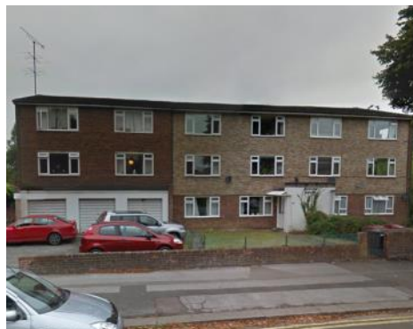
Shallow Pitched Roof & Brick
