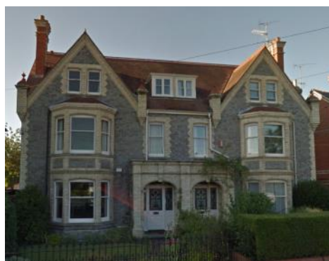
Elmhurst Road | Brickwork & Dormer
