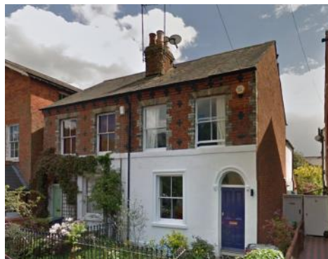
New Road | Render & Brickwork
