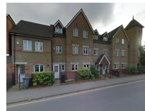
Christchurch Road | Brickwork & Hanging Tiles
