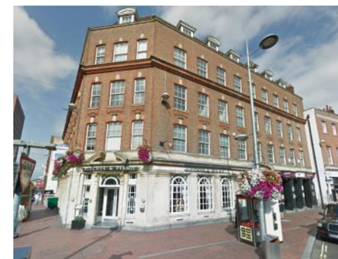
Station Road | Brick & Stone work
