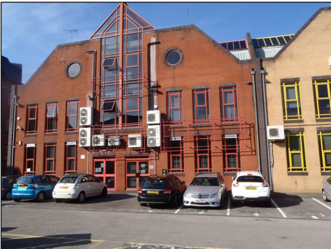
Rear elevation of 9 Southern Court (centre)
