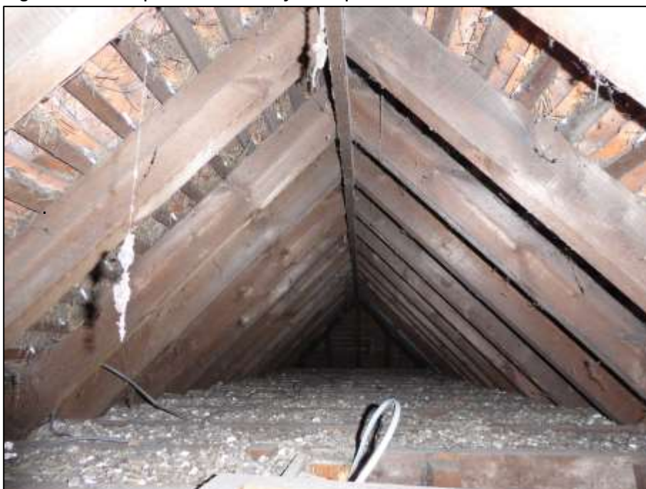
Figure 9. Example of subsidiary loft space. 11 Darell Road, Caversham.
