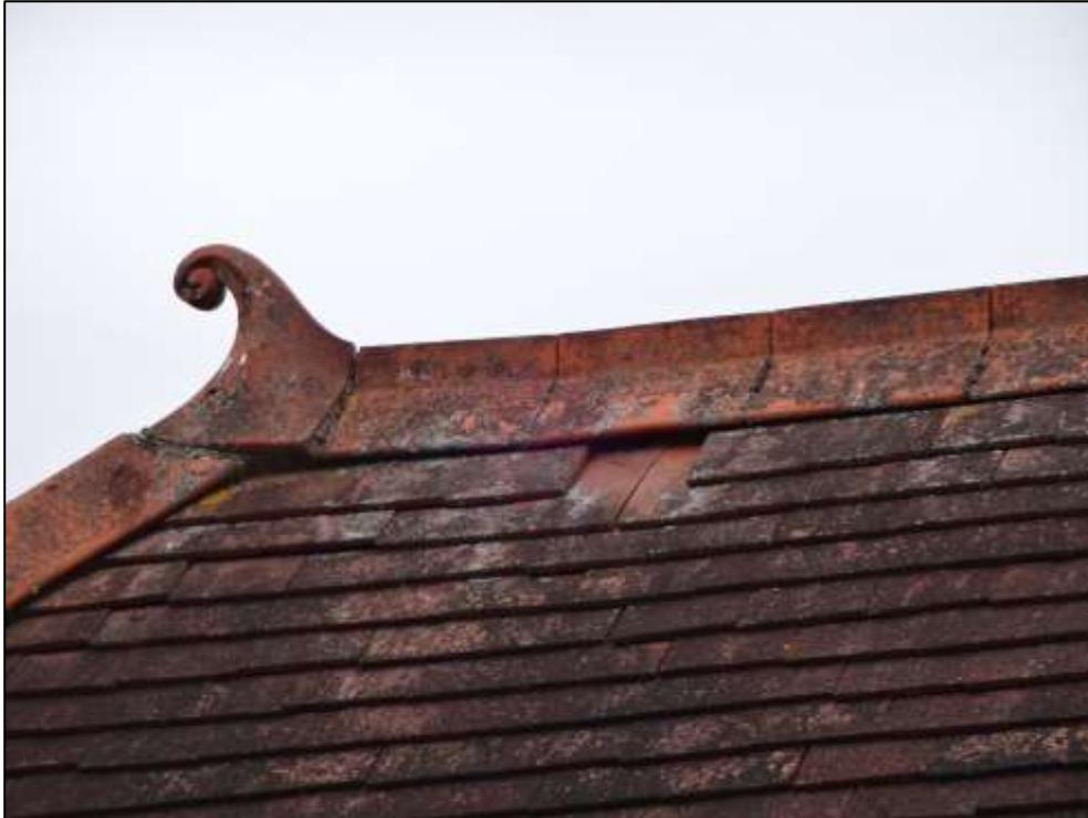
Figure 4. Example of gaps in ridge tiles, 11 Darell Road, Caverham.
