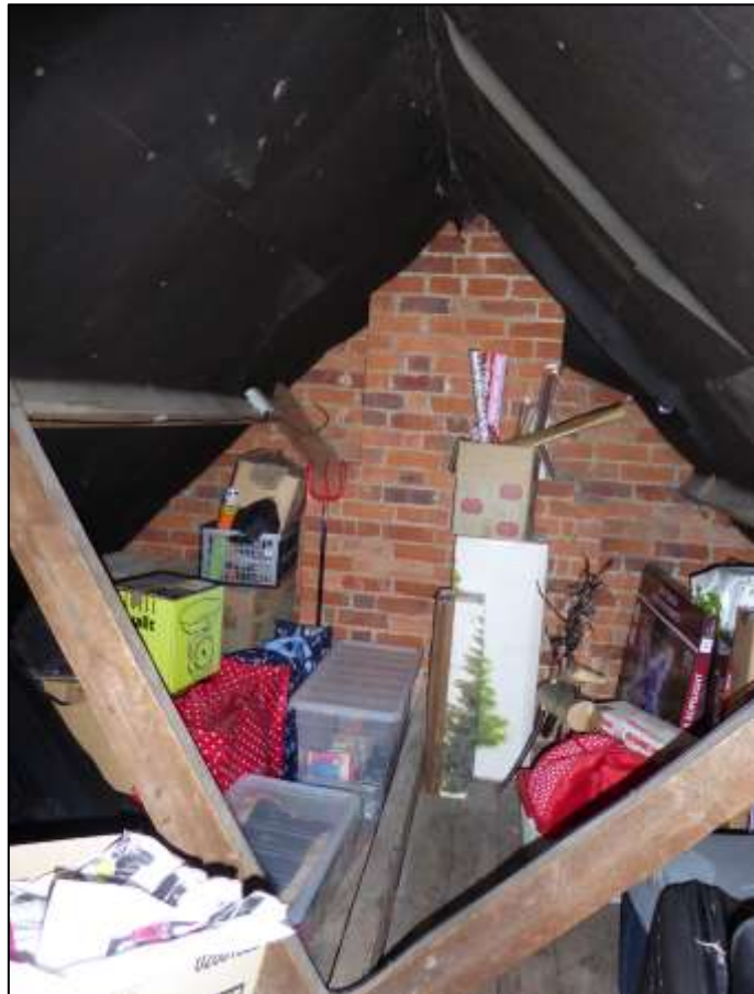
Figure 6. Example of unconverted loft space. 11 Darell Road, Caversham.
