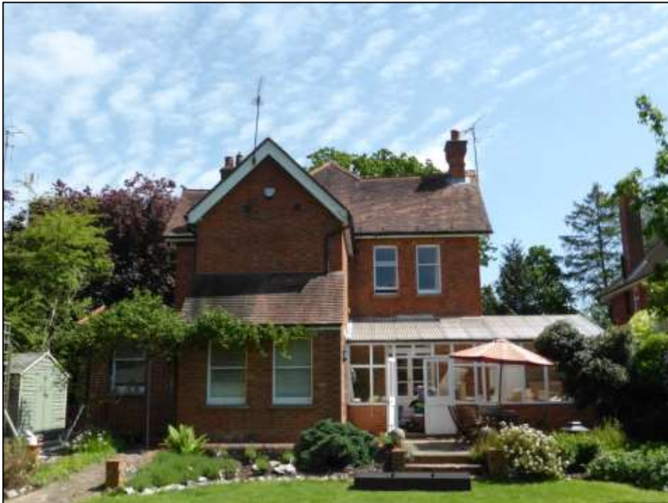
Figure 2. Rear aspect of 11 Darell Road, Caversham.
