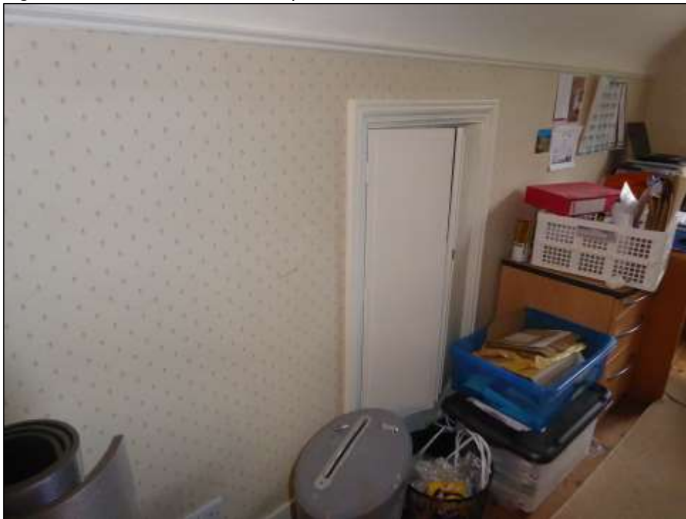
Figure 8. Access to eaves loft space, 11 Darell Road, Caversham.
