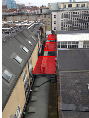
Existing plant decks to be reused
