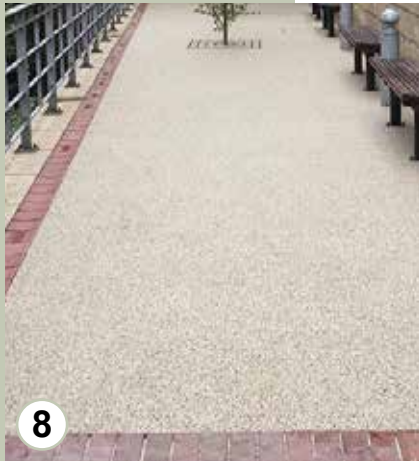
8 Amenity footpaths - East lake park Dekorgrip Resin Bound Gravel Pearl Grey 2-6mm aggregate laid at 16mm depth
