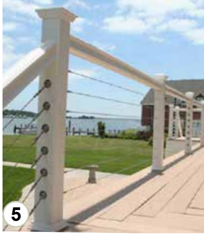
5 Timber top tensile wire balustrade Nautical fencing or similar 1300 mm high Stainless steel wires and stained or painted timber
