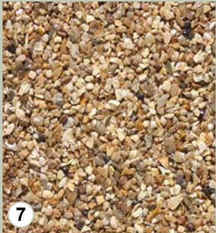
7 Ramp and pathway - East lake park Flexi-Pave Barnsley Solo Permeable aggregate 30 mm depth over MOT Type 1 hardcore
