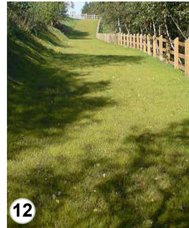
12 Emergency road North lake Grassroad or similar 42 mm depth on 150mm subbase
