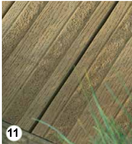
11 Footway board walk South lake Millboard composite deck Lasta grip Golden oak 200 x 32 x 3600 mm
