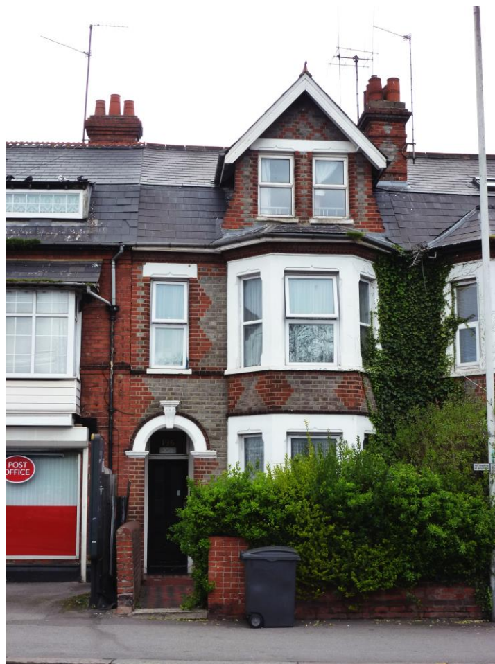
Fig.1: View of 196 Oxford Road from the street
