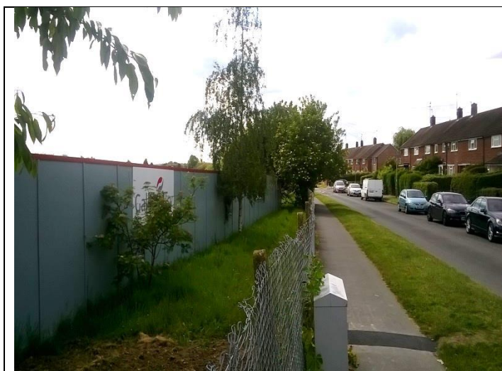
Site hoarding acting as tree protection.
