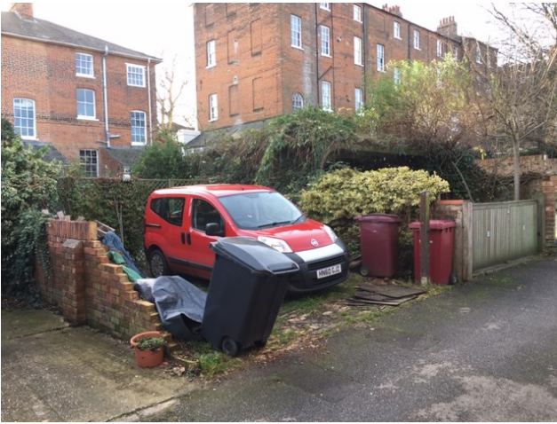
The rear of 142 Castle Hill, looking south west
