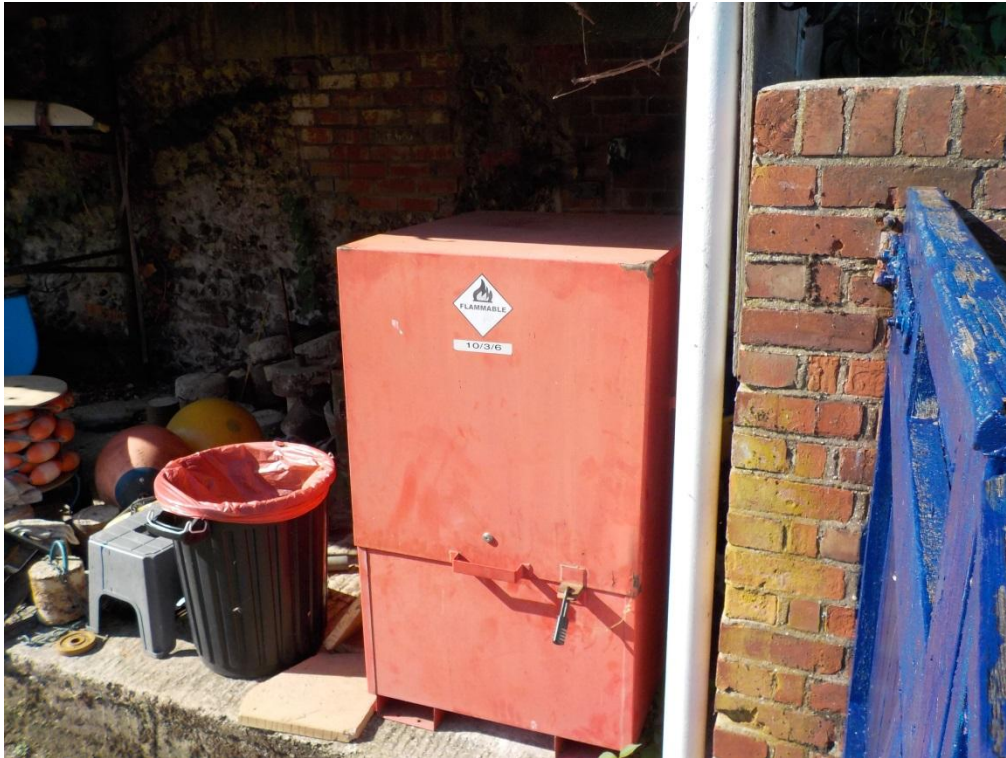
Plate 5: Flammables storage at The Dreadnought.
