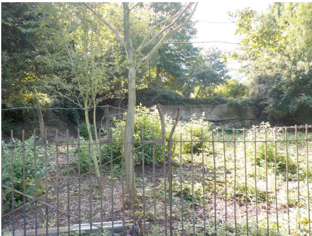
Plate 4: Retaining wall adjacent to the west of Wokingham Waterside Centre.
