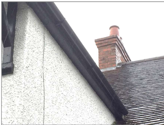
Photo 3 – Soffits on good condition
