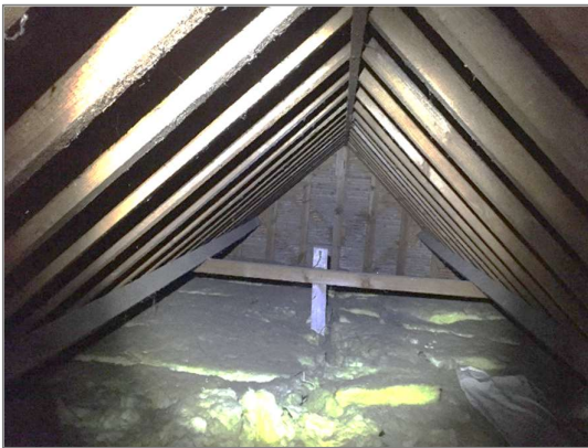
Photo 7 – General conditions of loft
