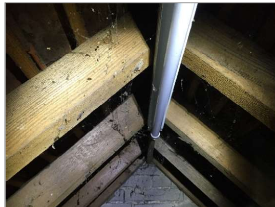
Photo 10 – north west gable apex
