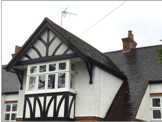
Photo 1 – Tiles to front of house
