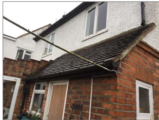
Photo 4 – Rear lean-to extension
