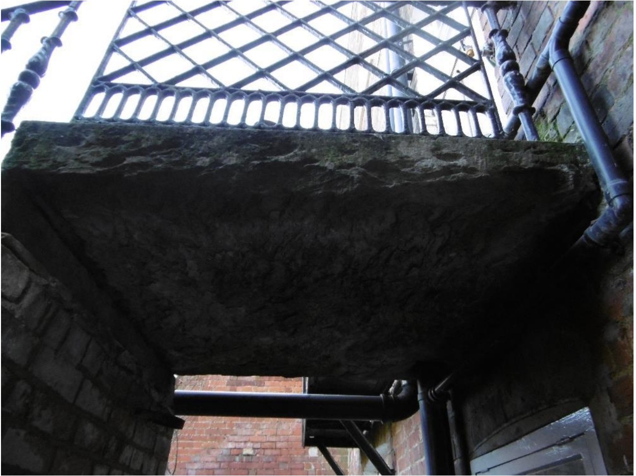
View on underside of landing slab
