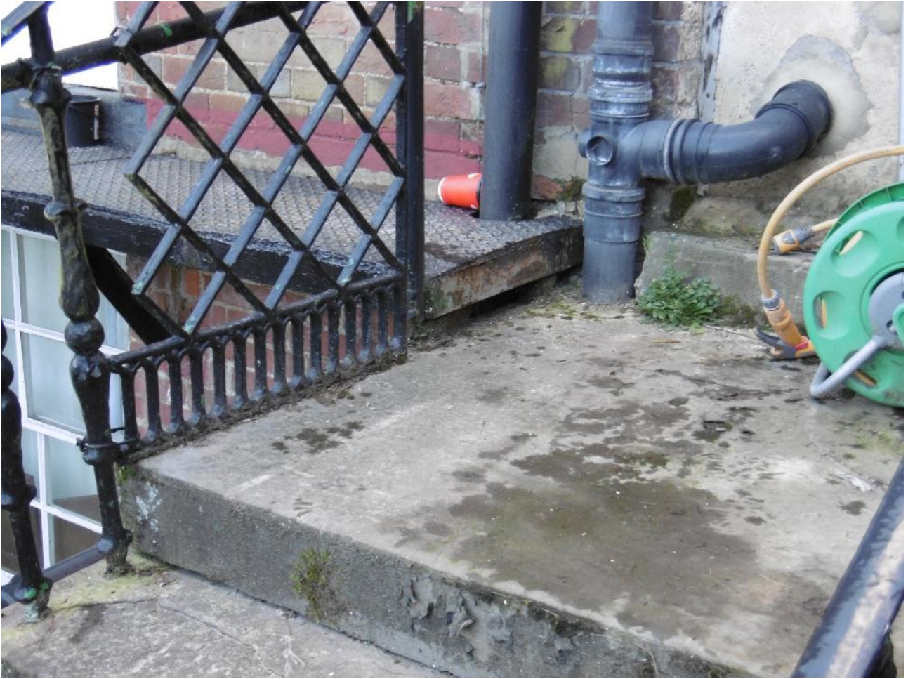
View showing balcony bearing on stone landing slab
