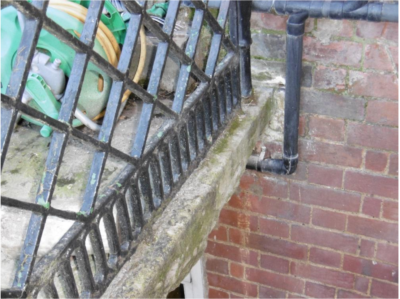
View on edge of landing slab
