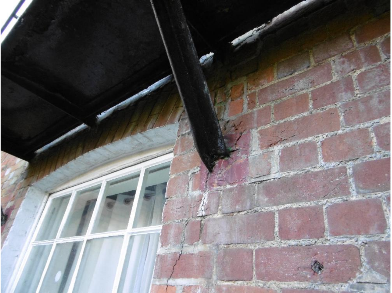
Close up view on bearing in external wall
