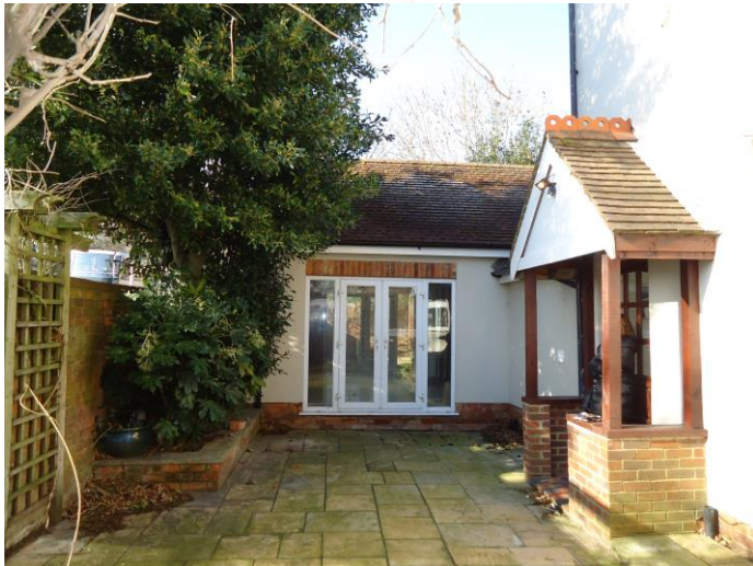
View from courtyard
