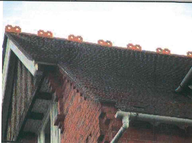
Detail of roof and front gable at No. 5
