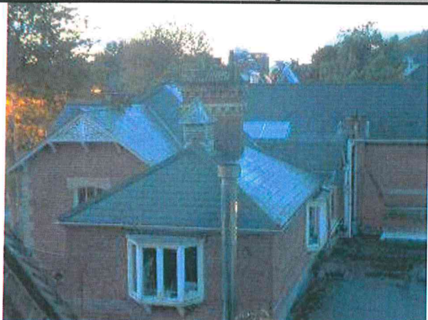
Central roof area linking the two buildings
