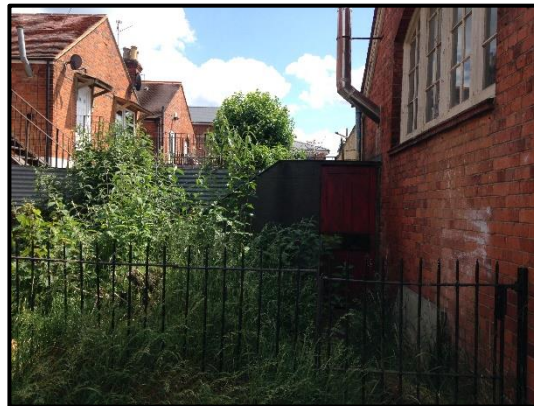
Photo 5: Cellar access which adjoins the Church Hall.
