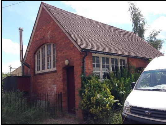
Photo 3: Church hall (west elevation).
