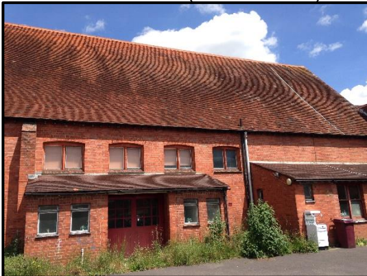
Photo 1: Church (south elevation).
