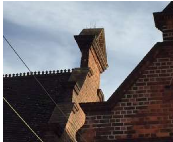
3 – Further high level brick parapets
