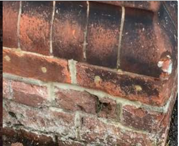
4 – Spalled brickwork
