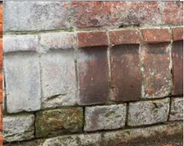
22 – Defective mortar
