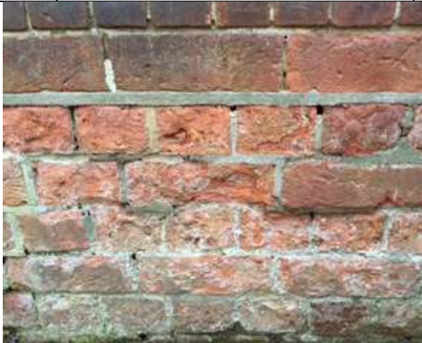
15 – Spalled brickwork
