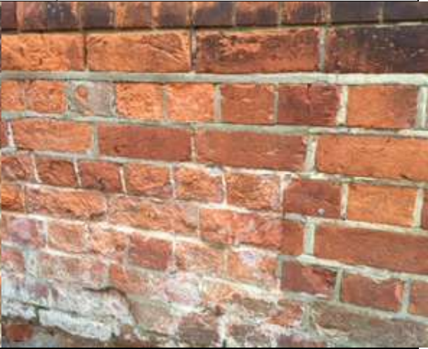
18 – Spalled brickwork
