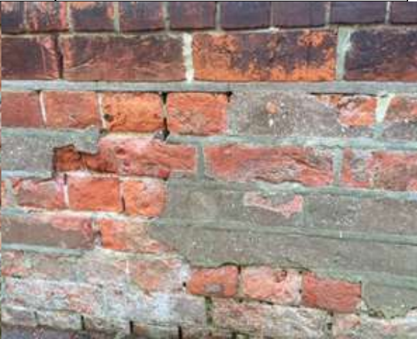
16 – Spalled brickwork
