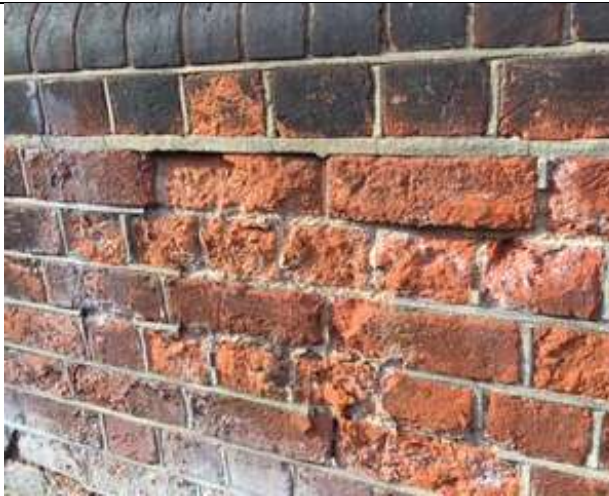
13 – Spalled brickwork
