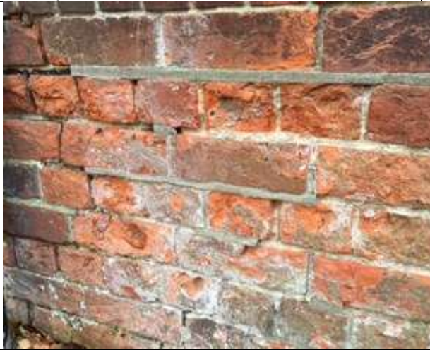
17 – Spalled brickwork
