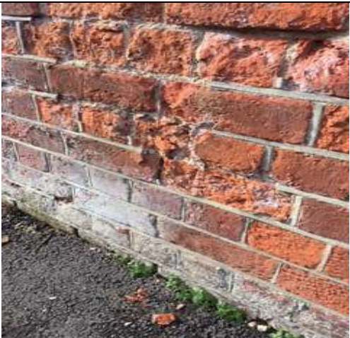
14 – Spalled brickwork
