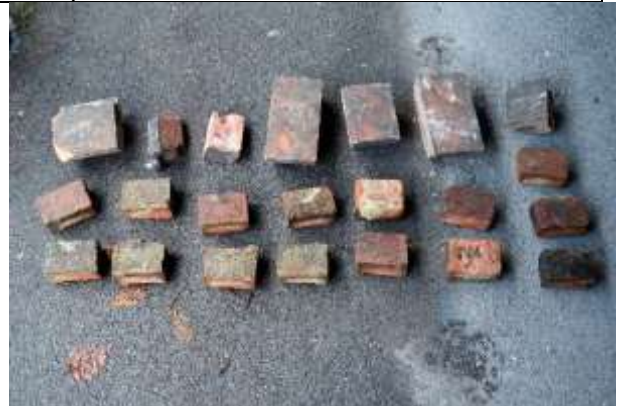
6 – Bricks that have fallen from height since June 2016
