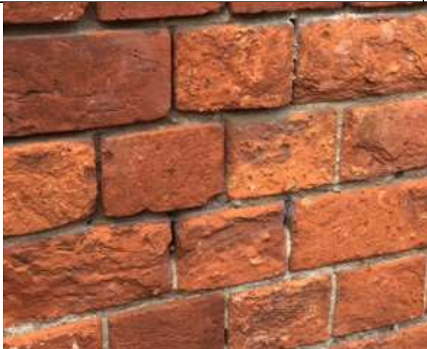
21 – Defective mortar
